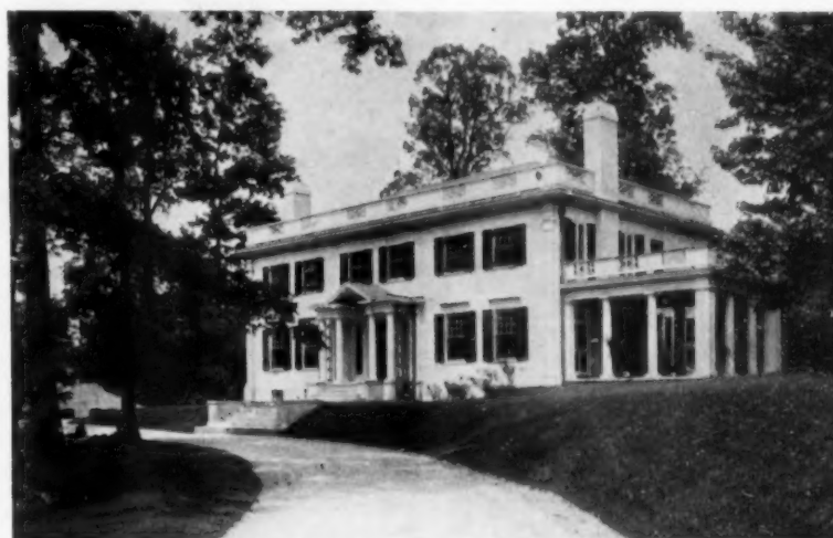
No. 8.—With equal effectiveness, this house could be built of white siding or shingles or all red brick
