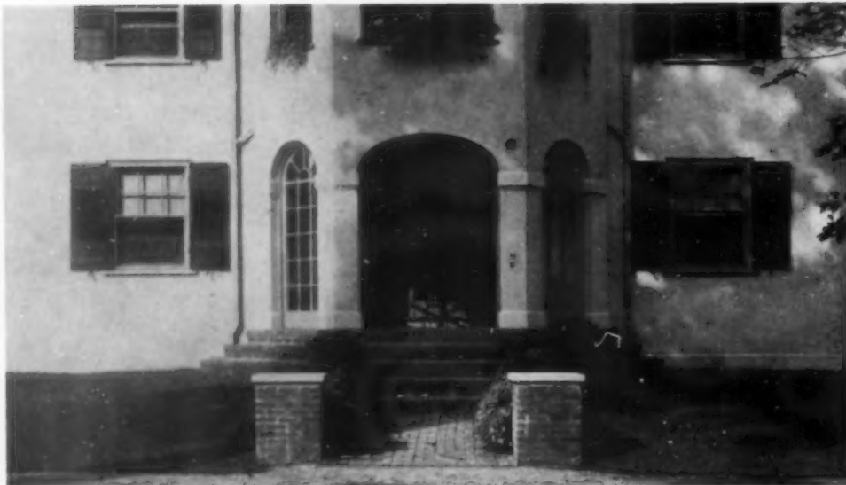
An entrance set inside a bay loggia with brick step and path giving approach. Here the lawns were also raised to conceal the height of the first floor above grade at the front
