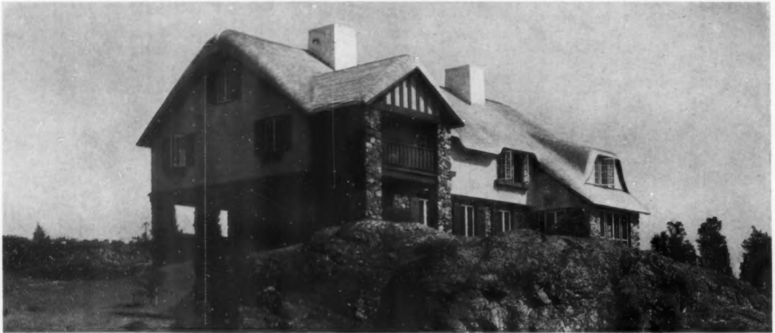
Wall construction in this house at Marblehead was a deliberate effort to suit the setting—rough fieldstone laid in open bond tones in with the rocky foreground; vertical half-timber following lines of nearby trees; and the remainder stucco, a reproduction of the generally unobstructed atmosphere about the house. Charles M. Baker and Allen W. Jackson, associate architects
