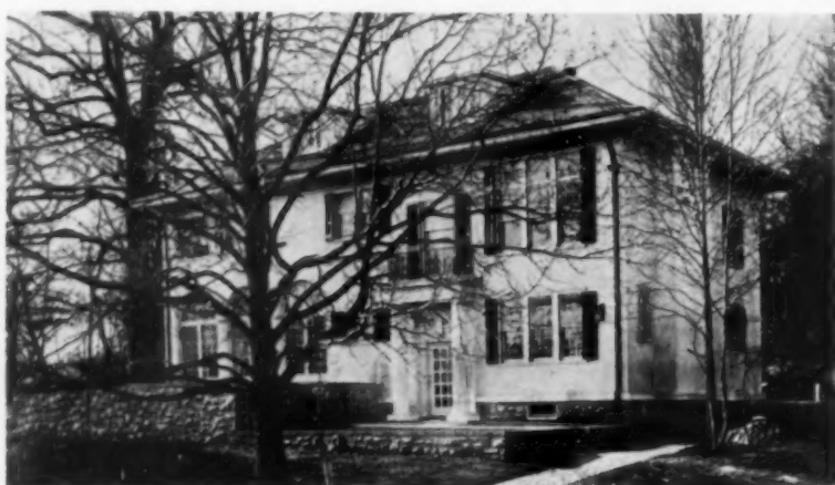
No. 3.—An unbalanced formal type of white stucco. The interior arrangement shows rooms at different levels
