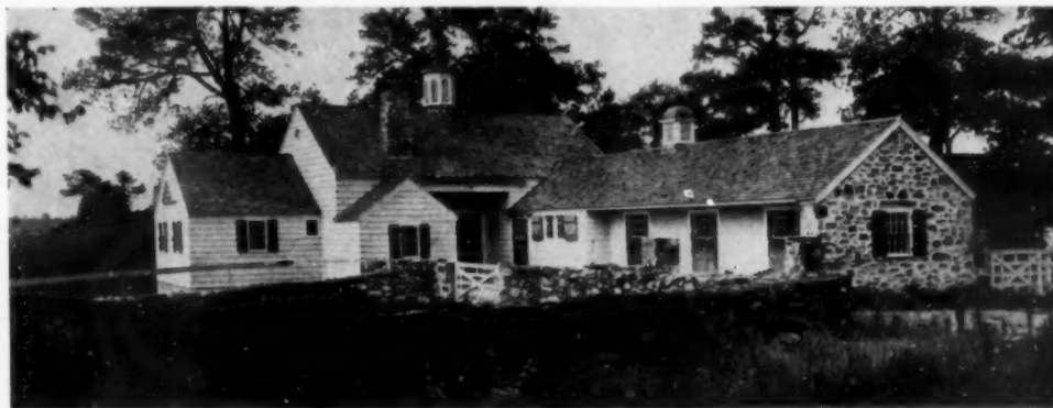
Two types of walls used successfully in a farm building—shingle with an end wall of field stone that "ties up" with the roadside and stableyard walls
