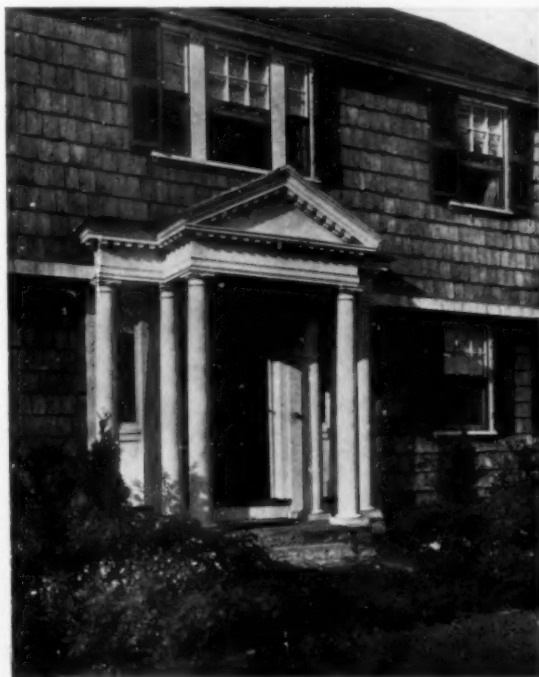
Uneven and rough as hand-split shingles may be, they weather well and lend an air of distinguishing artistry to a house
