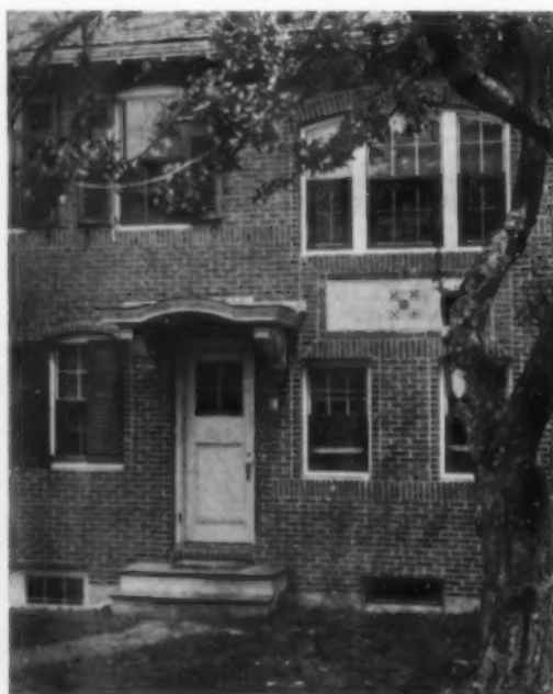
The side door can also be made distinctive if hooded in some such manner as this
