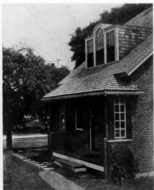
A service entrance saved from banality by a hood, an extension of the roof
