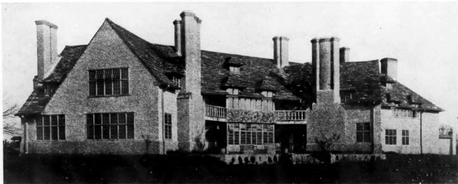
An English house where the physical form of the roof line eliminated all but one type of material—heavy slates laid irregularly. As a study in the skyline the house it presents some interesting points, a logical outcome of the rest of the structure
