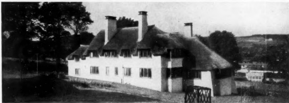
Thatch is often used on modern houses in England with excellent results. When well laid it is no more inflammable than shingles and is impervious to the weather
