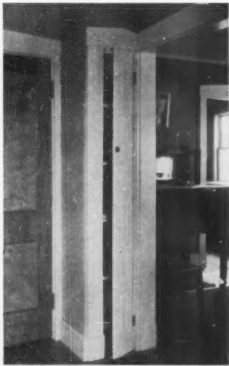
Where the thickness of the partitions allows it, such a handy closet can be built in
