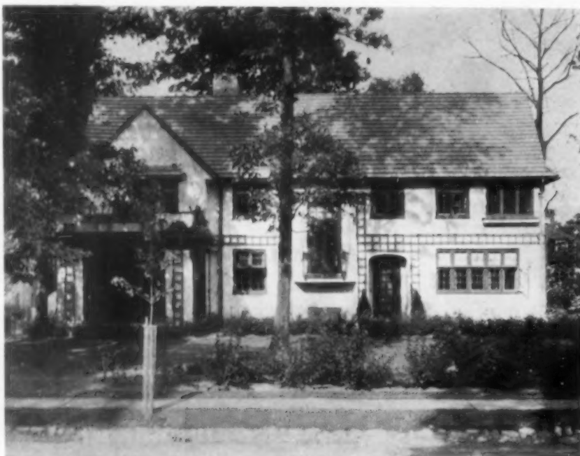
No. 4.—The general use of mullioned and transomed grouped windows suggests the rural English type. A house that could also have a brick and stucco exterior or half-timber and stucco
