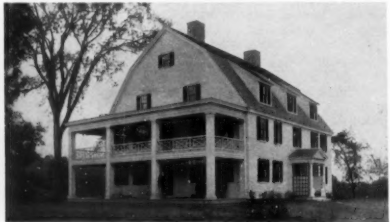
All-over clapboard walls in a Dutch Colonial house where simplicity of wall treatment was most desired
