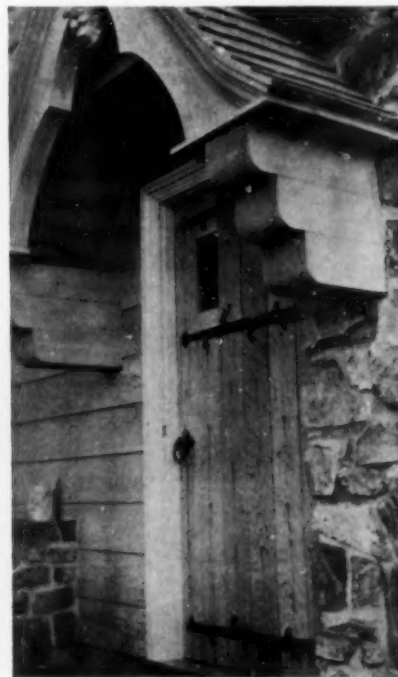
Where field stone and clapboard meet the connection can often be effected through the medium of a heavy, rough door
