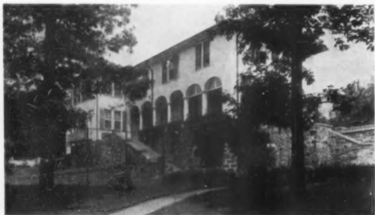
No. 2.—A house on a hillside planned along Italian lines, a type permitting an irregular arrangement of rooms
