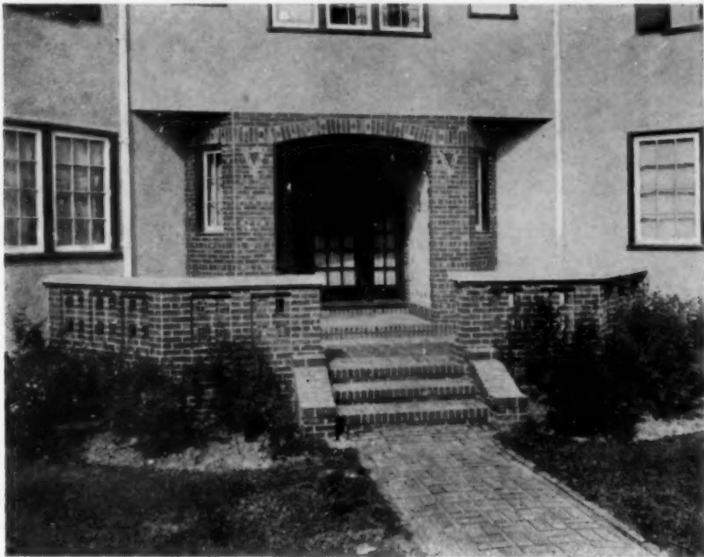
Privacy lent a doorway recessed within a protective vestibule. Here the horizontal lines of terrace and step also produce an approach that overcomes a heavy rising grade
