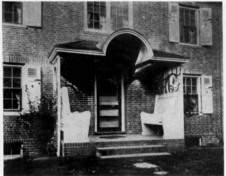
Modesty of line and construction characterize the details of this cottage Colonial entrance. The hood seats and lattice are tied together in one congruous whole, to be further enhanced by vines
