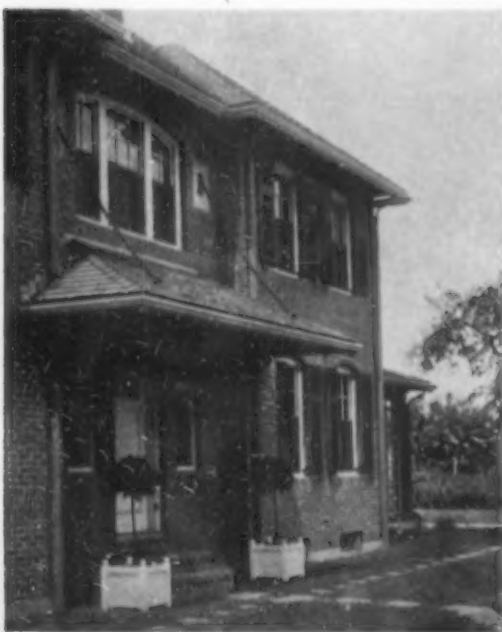
An effective treatment for a suburban brick house—a hung front doorway hood
