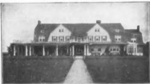
Residence of Ralph Peters, Esq., President Long Island R. R. Aymar Embury, II., Architect, New York Shingles stained with Cabot's Shingle Stains, stucco stained with Cabot's Waterproof Cement Stains, and lined with Cabot's Quilt for warmth
