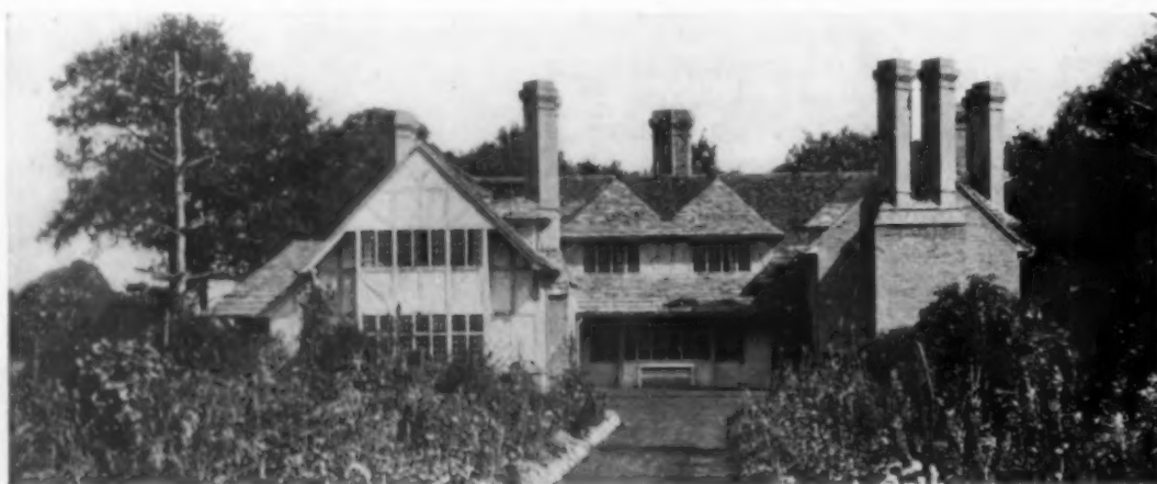
Slate is used effectively on the roof of this English country house, the roof lines of which, characteristically British, might serve as a model on this side
