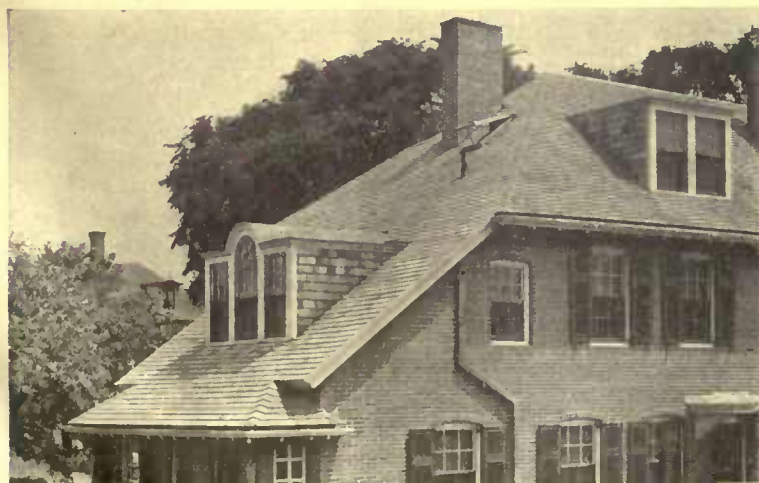
A mottled effect produced by unstained shingles allowed to weather for a time is attractive
