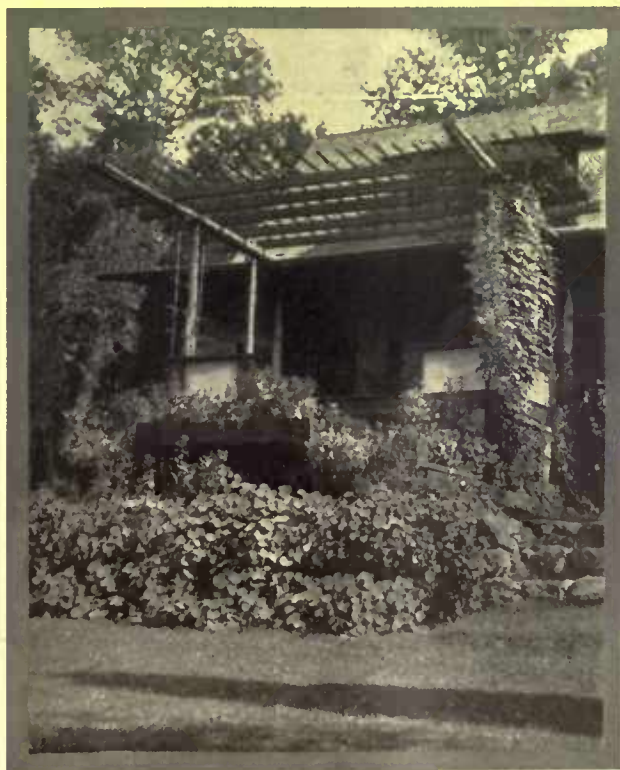
Instead of the conventional awning a pergola-like roof was formed of lath. Over this vines were trained
