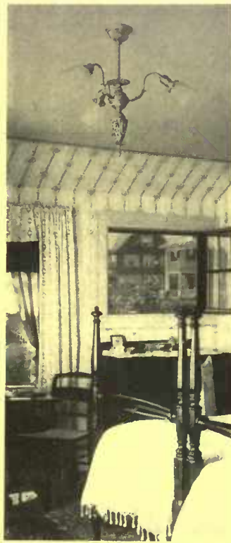
Fixture arms at this angle are incorrectly placed; the globes expose the lamps
