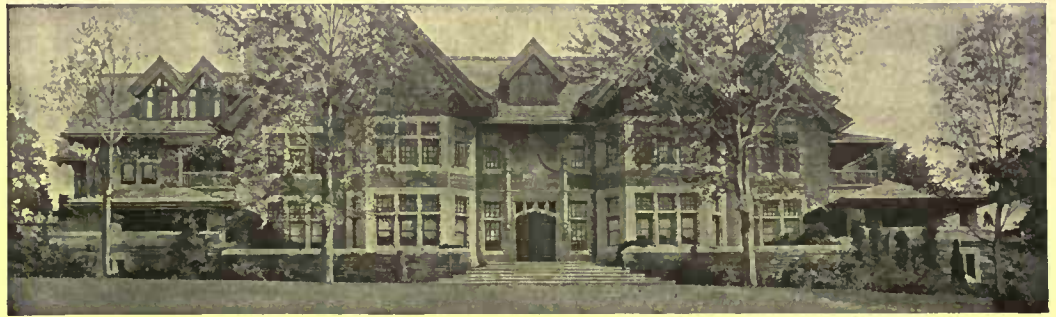
Residence of Dr. George Woodward, St. Martins, Pa. Peabody & Stearns, Boston, Mass., Architects
