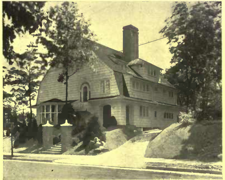
When the house must be close to a street, have the entrance porch small and let the true piazza features face on the land
