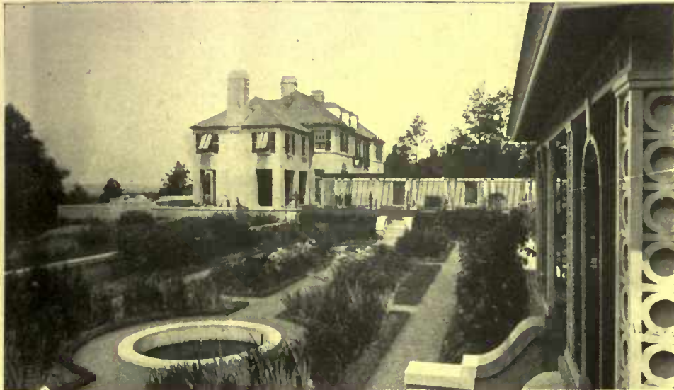
From the extreme end of the lower garden one looks toward the loggia and the upper garden with its pergola-covered walk. This view shows the disposition of the most important rooms to take advantage of the attractive view to the west
