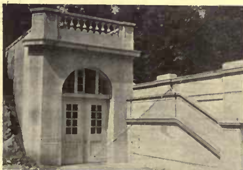
A small, formal garage of reinforced concrete construction
