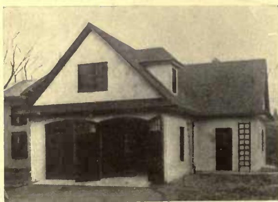
A good fireproof brick and stucco type having a shop on one side
