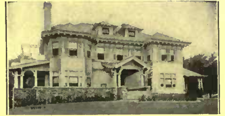
Residence of C. B. Manville, Pleasantville, N. Y. Covered with J-M Transite Asbestos Shingles. Betts & Hosmer, Architects, Milwaukee, Wis.
