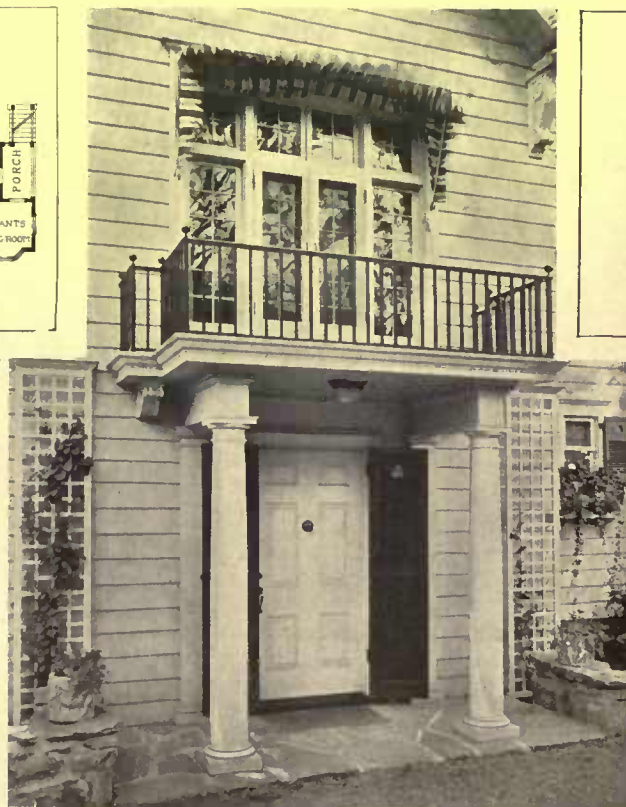
The driveway entrance is unpretentious but attractive. The broken stone flaggings is a fitting feature in this situation
