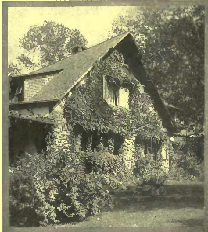
The windows instead of being separated were grouped in most cases, and each room had light from but one direction
