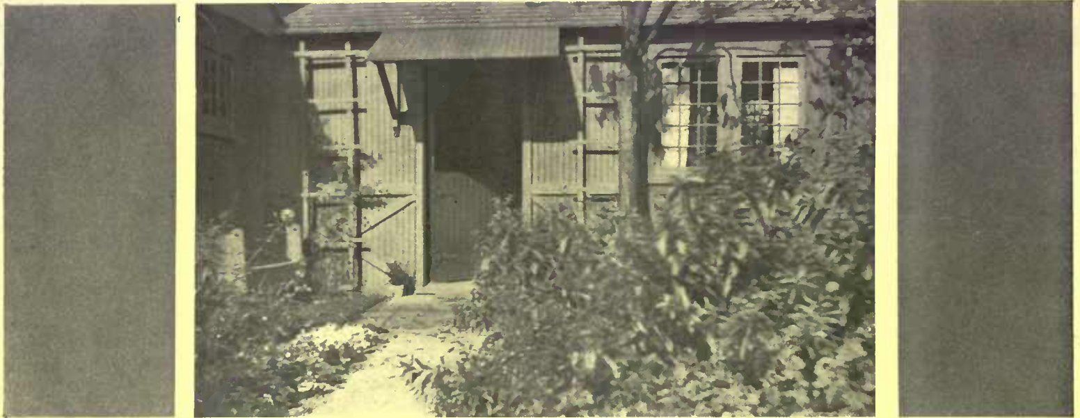
The addition of an old Dutch door and knocker, trellises for climbing roses and ampelopsis, and casement windows in place of the original small lights, transformed the building
