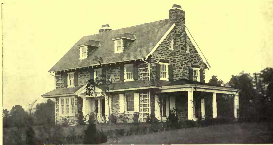
The house of rough stone, however substantial its exterior may appear, must have very thick walls to insure warmth
