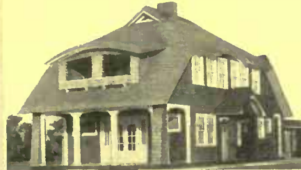
"CREO-DIPT" Shingle Roof and Side Walls. Freeburg & Fidler, Architects, Jamestown, N. Y.
