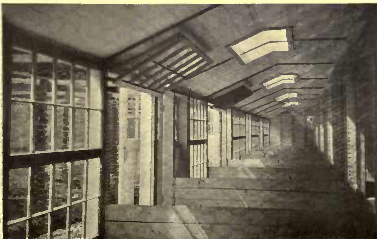
The large windows fold in the center and may be hooked against the ceiling when more air is desired
