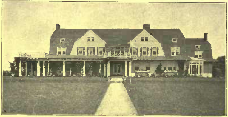
Residence of Ralph Peters, Esq., President L. I. R. R. Co. Aymar Embury II, Architect, New York. Shingles stained with Cabot's Creosote Stains; Cement stucco stained with Cabot's Waterproof Cement Stains; Walls lined with Cabot's Quilt for warmth.
