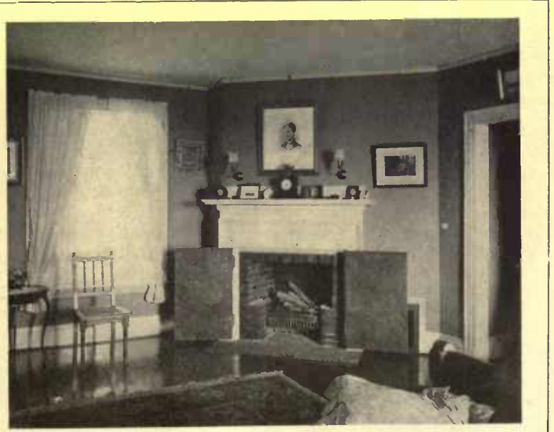
The annoyance of drafts from the fireplace may be remedied by hanging two doors such as shown in this illustration
