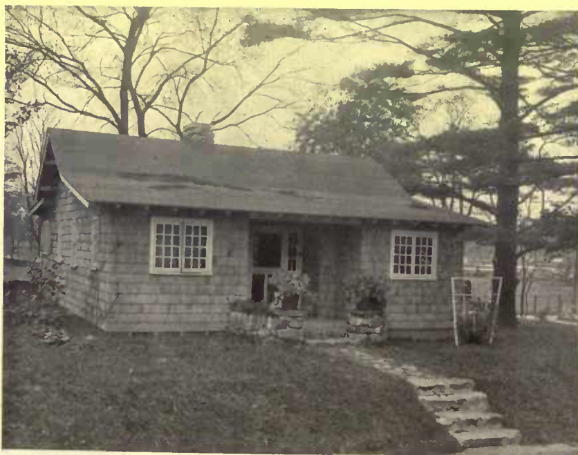
The shingled wall type is appropriate in certain locations. The roof in this case is papered throughout
