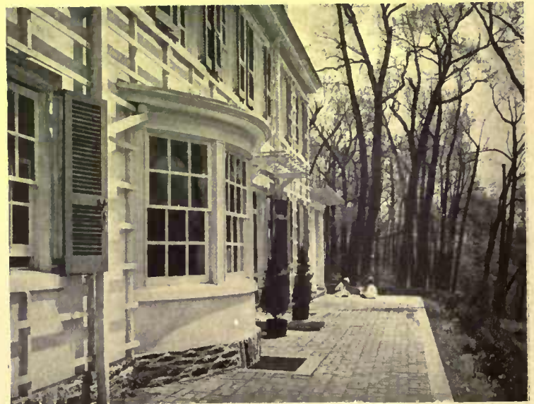
The wide eaves over the windows are distinctive and the red brick tiles contrast well with the gray underpinning and white plaster walls
