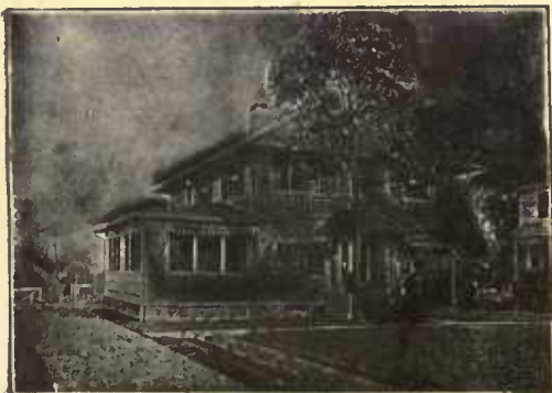
Residence of J. L. Johnson, Esq., Hackensack, N. J. Menn & MacNelle, Architects, New York
