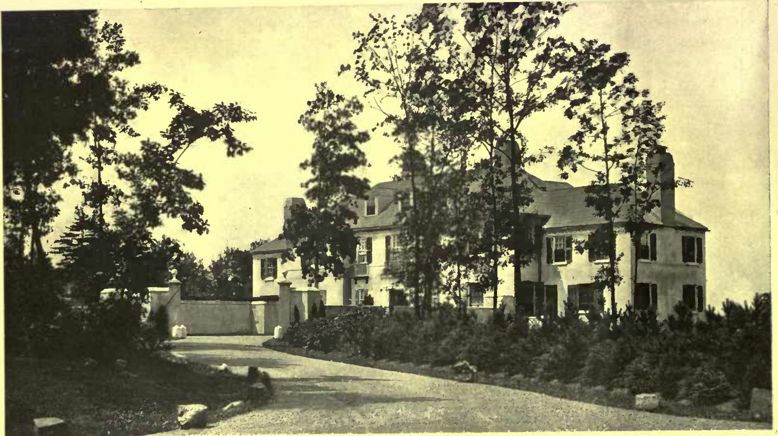
The claim that a perfectly symmetrical house is cold and stiff is not substantiated by fact, since the placing of the house in its site has much to do with its impression of attractiveness. Seen from the driveway this residence appears inviting
