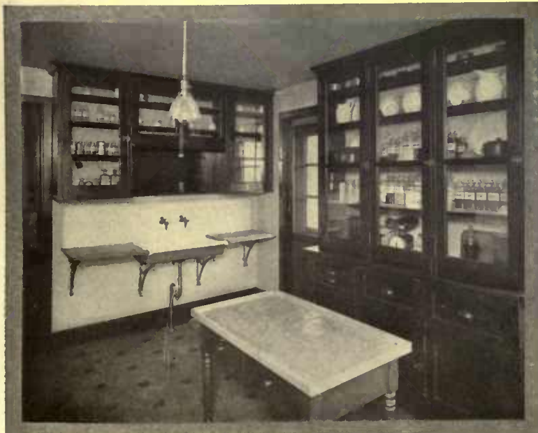
The most approved kitchen sinks have the body, back and drain shelf all in one piece. This is a desirable fixture, very simple in its drainage and faucet equipment
