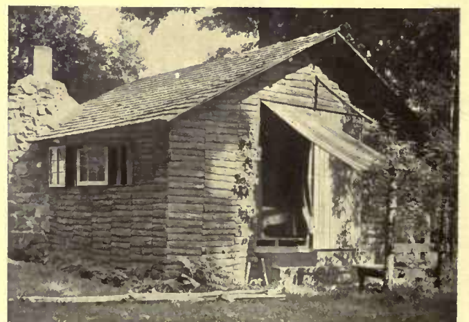
In this four hundred and fifty dollar bungalow sheathing boards overlaid with bark conceal the frame building
