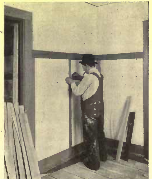
The various sorts of plaster or composition board are a reasonable and efficient substitute for plaster. They may be applied directly to the studing and if battens are used over the joints, successful approximate paneling is realized. They are ready for use and need only painting, but the directions for cutting should be carefully followed
