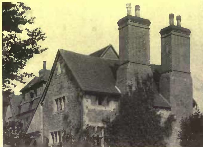
The slight irregularity in the laying of the old tile roof produced interesting texture effects
