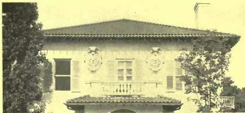
The appearance of a tile roof is improved when the various tiles are left open at the eaves, producing the interesting wave line
