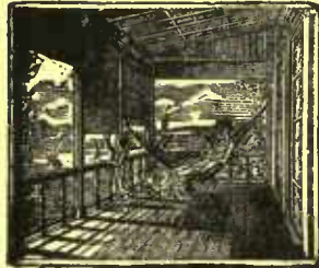
Wilson's Porch and Piazza Blinds
