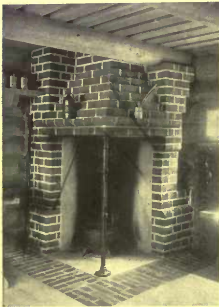
Fireplaces are located in corners, an iron support serving the purpose of a crane
