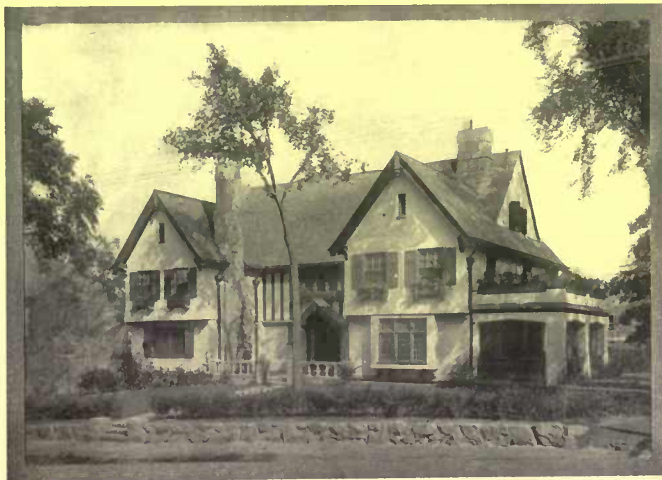
This house has a variety of elevations without extreme irregularity of plan. The porch roof provides a possibility for a sleeping porch with iron awning supports as suggested
