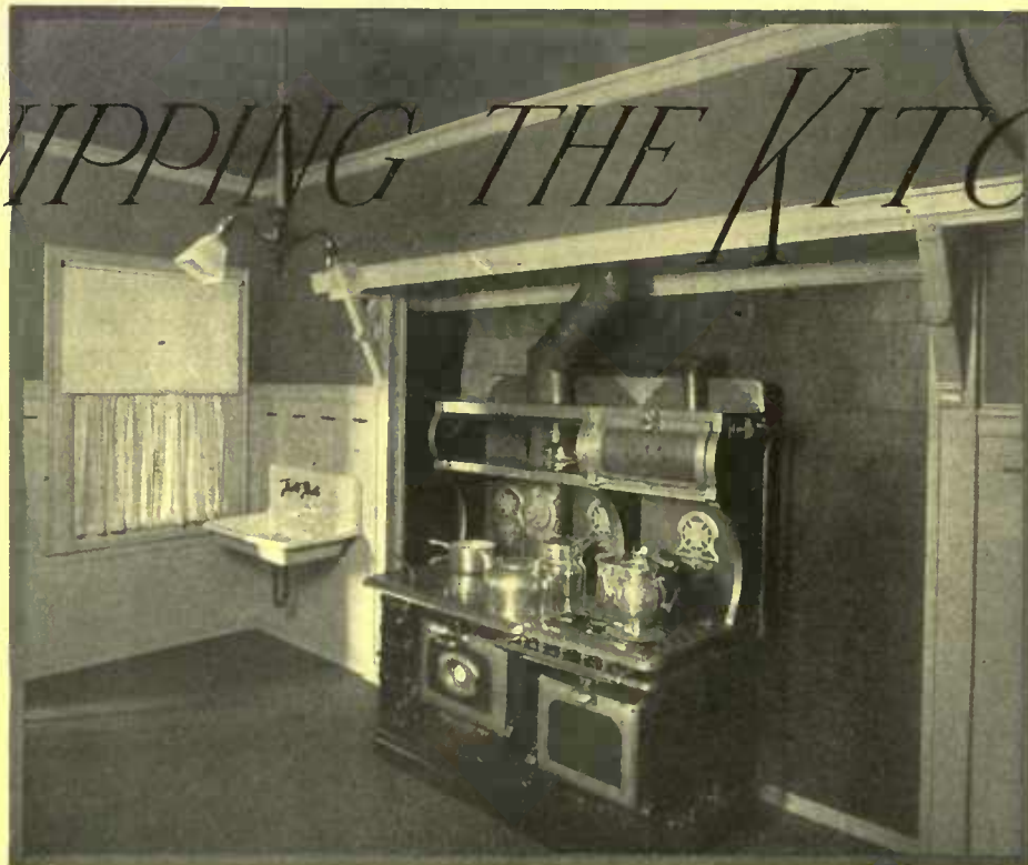
A shallow alcove designed for the range and lined with tile or brick saves space in the small kitchen and does away with smoke and cooking odors
