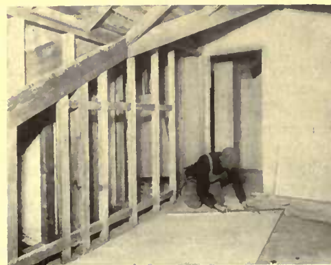
The various sorts of plaster or composition board are a reasonable and efficient substitute for plaster. They may be applied directly to the studing and if battens are used over the joints, successful approximate paneling is realized. They are ready for use and need only painting, but the directions for cutting should be carefully followed
