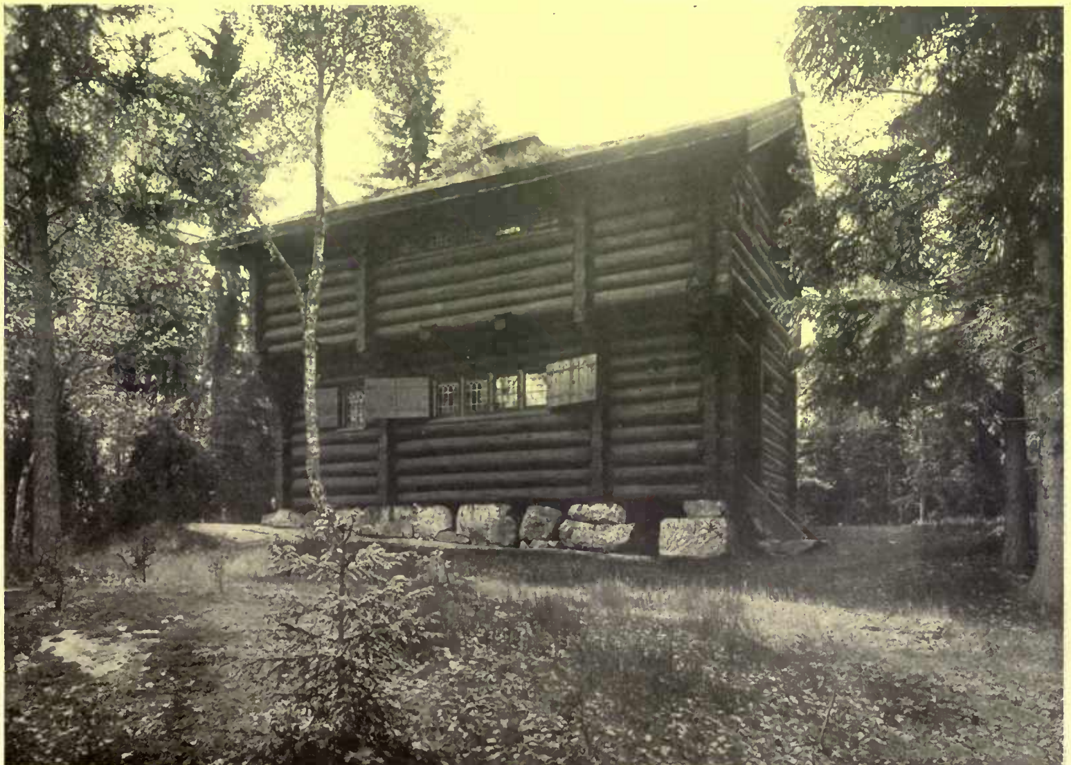
There is no excavated foundation to the log cabins of Sweden, but the house rests upon the ground and a foundation of heavy stones. The leaded windows with solid shutters are characteristic. Nearly all the partitioning is structural, as may be seen from the log ends projecting at either side of the row of windows
