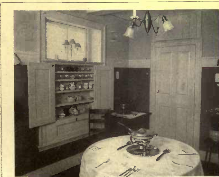
A unique way of replacing the buffet by a cupboard in the wall. This arrangement saves valuable space
