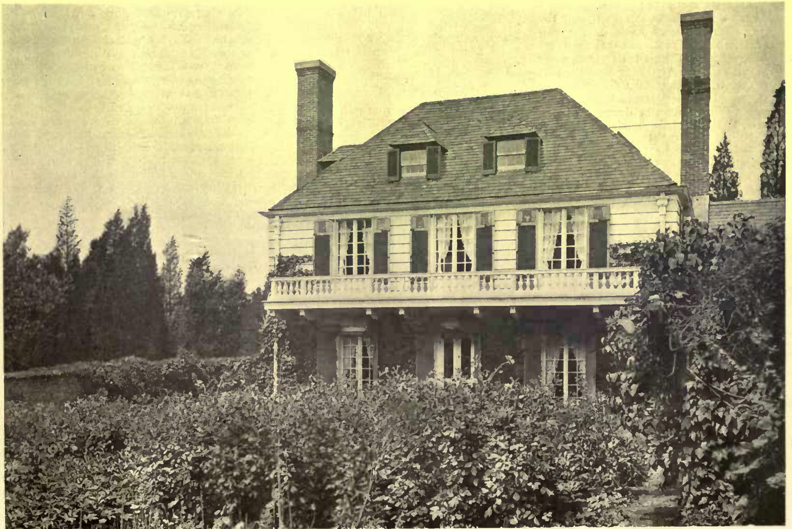
A garden wall forms an elbow at either side at the rear of the house enclosing a luxuriant growth. The French windows and the door open directly on the garden and a balcony overlooks it, making it seem another addition to the rooms. The balcony on this side is distinctly interesting
