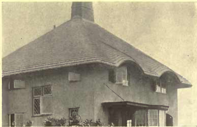
The use of shingles may be varied to produce pattern effects of various lines such as is shown here
