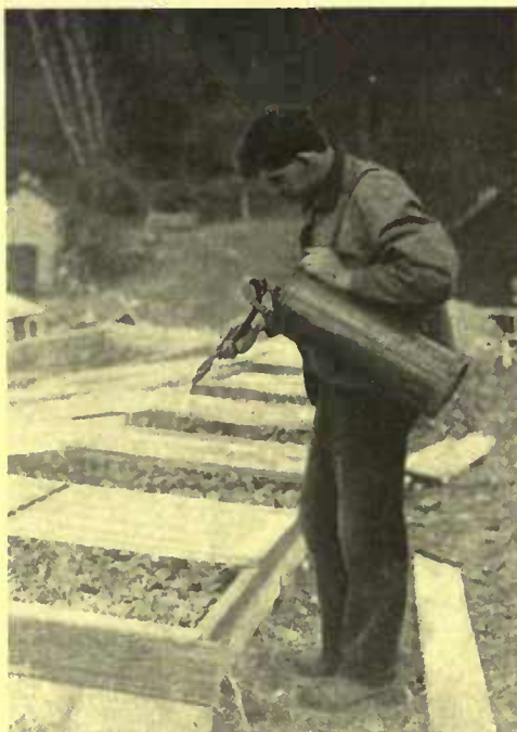
The compressed air sprayer is charged with a few strokes of the plunger, hung from the shoulder by a strap, and is ready for use
