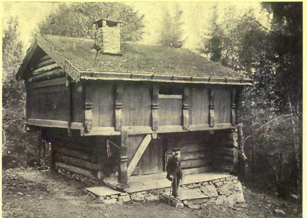
A very ancient log cabin that shows the possibilities of timber decoration. Here boards are substituted for the logs in the second story. The roof shows the means of keeping the sods in place
