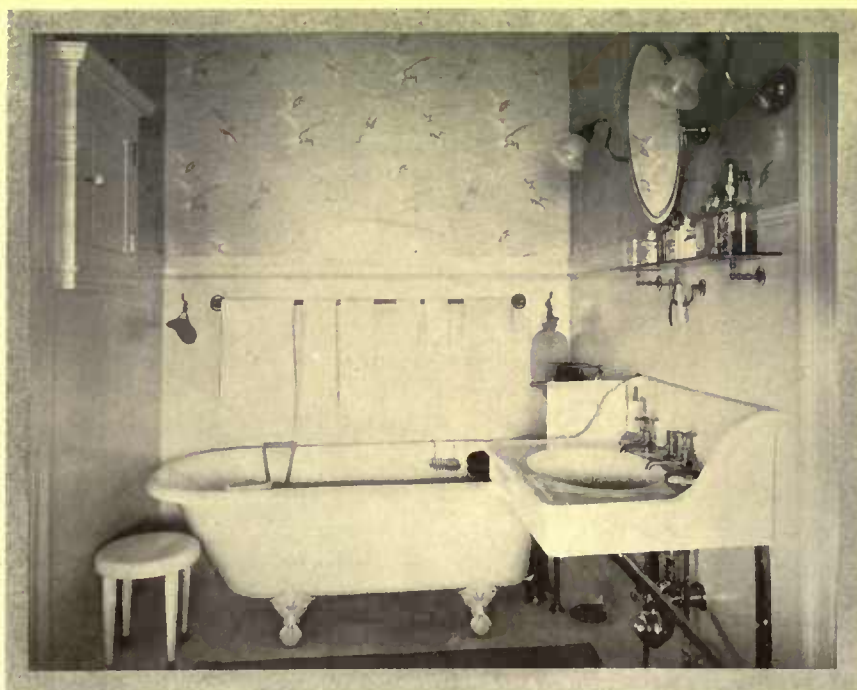
A modern bathroom showing how the visible piping is restricted to but a few lengths of pipe, and this made attractive with nickel fittings and beautiful finish
