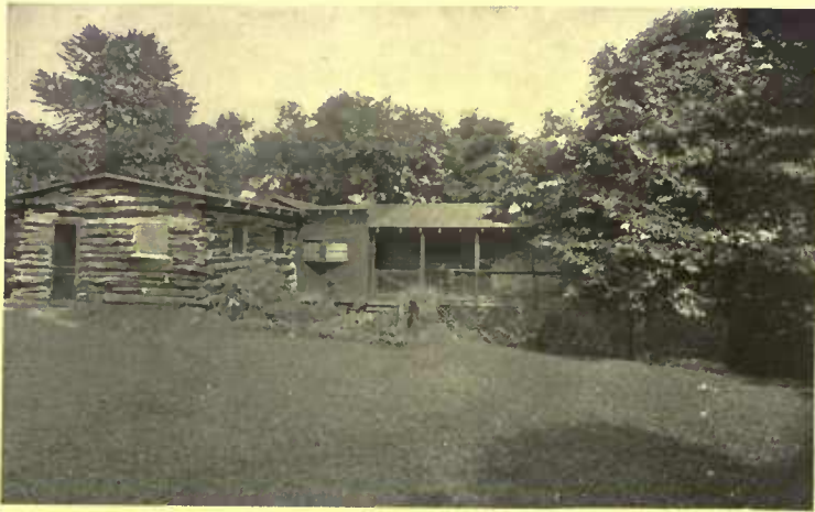
A log camp in which the space below the veranda wing, caused by the sloping ground, is latticed and used for storage purposes
