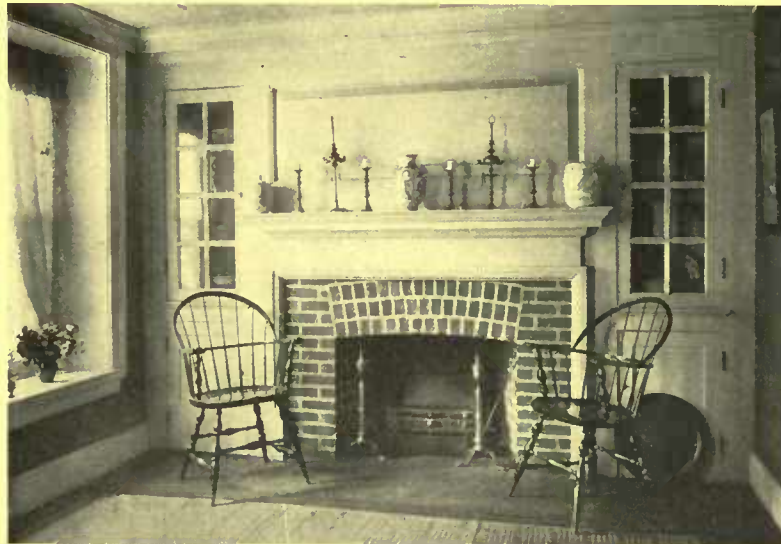
Ugly and useless chimney space can be eliminated by a symmetrical arrangement of cupboards
