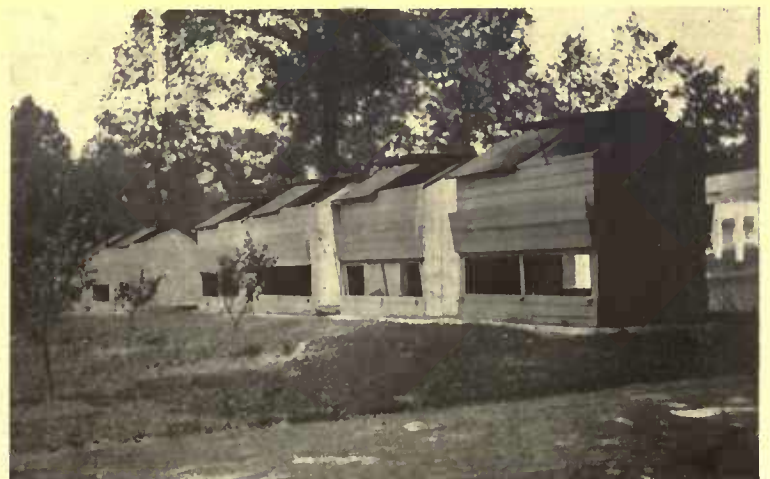
A good type of colony house for permanent location showing the method of raising the hinged roof
