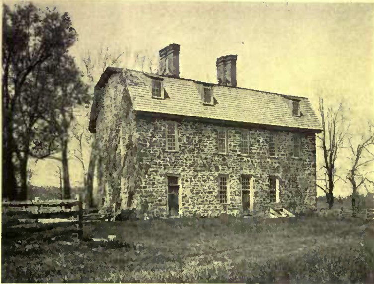
From the rear is shown an interesting adaptation of the gambrel roof to a house that is narrow in proportion to its length
