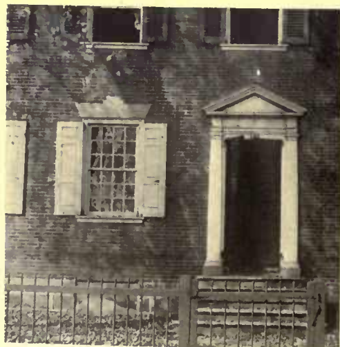
A typical Colonial window of 1770, with small panes and a "Jack-arch" head
