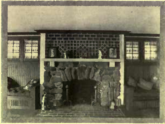
The fireplaces showing an effective use of tapestry brick in combination with stone
