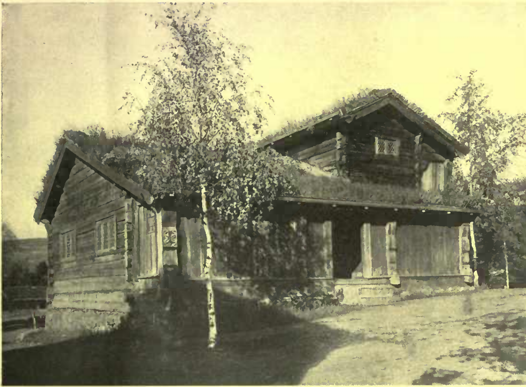
The roof is covered with turf or sods which by a judicious use of building paper is weather-proof and lasting. The grass and blossoms grow to give a very beautiful effect
