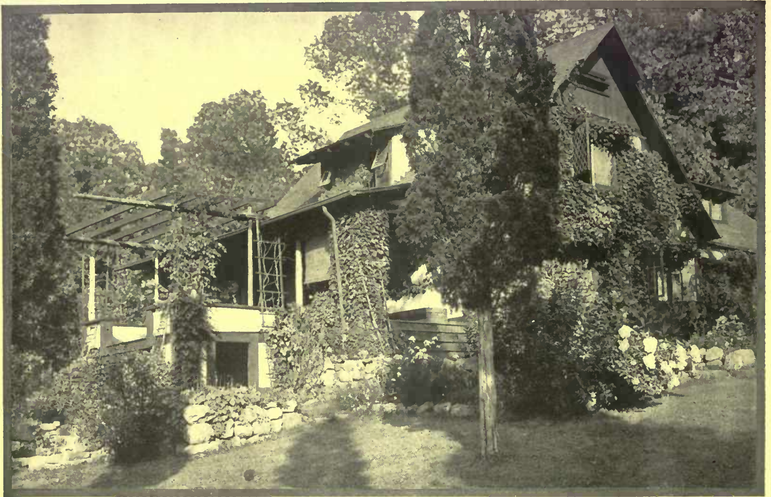
From the idea of the mountain house which fits so snugly into the countryside the design was chosen. By proper planning eight-foot railroad ties served for most of the timber and the stone work was taken from an old wall
