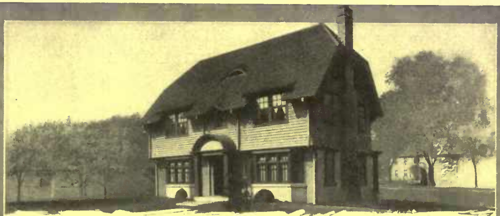
Residence of Mr. J. B. Thomas, Elyria, Ohio. John Henry Newson, Cleveland, Architect. A Pierce-American Hot Water Boiler provides ample heat with the minimum of attendance and expense.
