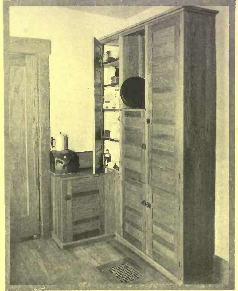
The built-in cabinet gives opportunity to carry out individual ideas. It should have shelves of varying height and bins for flour
