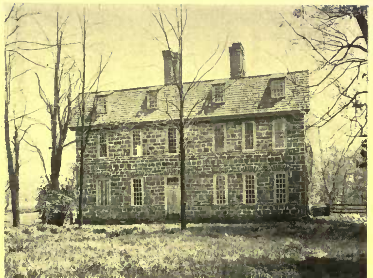
Between the two rows of narrow windows are courses of shaped stones that offer a pleasing variety in the design
