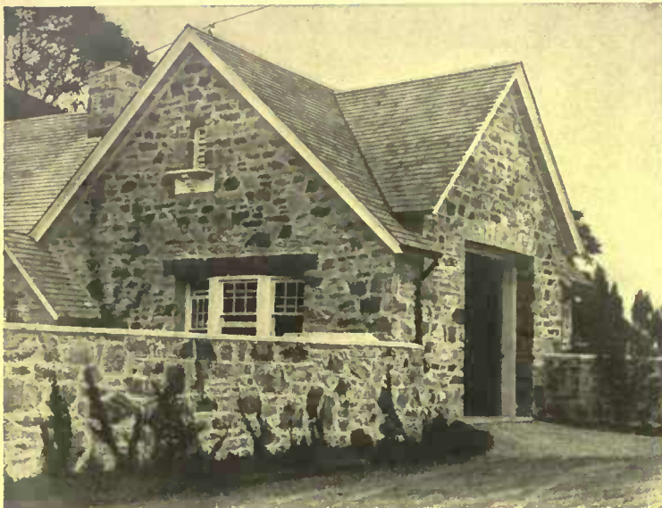
The stone garage has the advantage of being more fireproof than one of frame construction, and it often has greater architectural worth
