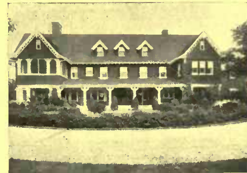
Residence of H. Cart Johnson, Millneck, N. J. Heated by Kelsey Warm Air Generator.
