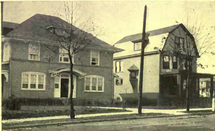
The right-hand house is a meaningless hodge-podge of bays, casements and dormers; the other has its windows carefully spaced and proportioned
