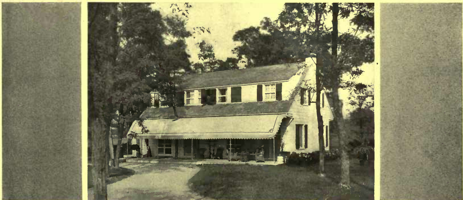
A cottage that provides porch shade without an excessive roof overhang. James W. O'Connor, architect
