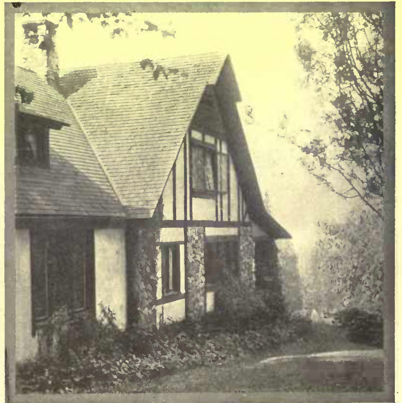
The half-timber work was of the sort used in the English houses; that is, was structural rather than purely decorative
