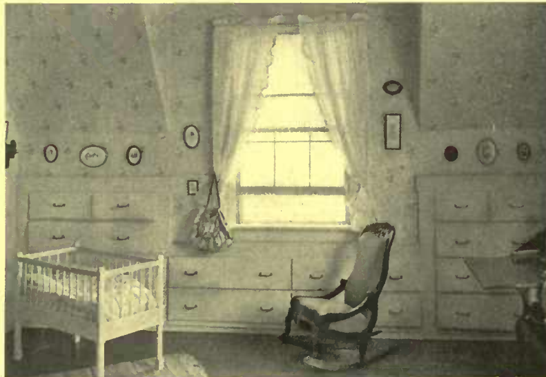
Chests of drawers built into sloping roofs around dormers utilize waste space and remove the unsightly slope of the eaves
