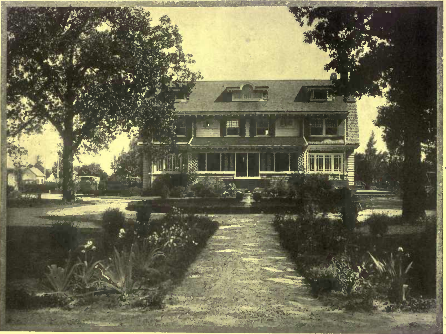
The Rhoads house does not front upon the street, and obtains privacy thereby, the entrance stairs being upon the side and through a porch that may be inclosed. The gambrel roofed type was utilized here for the coolness obtained by projecting eaves, the windows of all the main rooms on the south side being shaded
