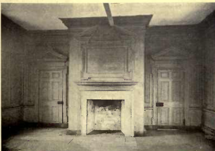
Fine Colonial detail is evident in the rooms, especially about the great fireplace and mantel and in the wainscoted walls
