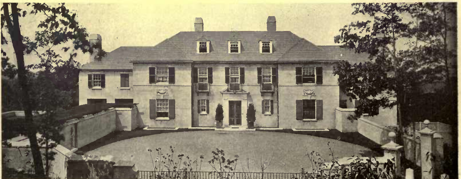
A circular turnaround inclosed with a wall is at the east front of the house. At the left the wall forms a basis for a pergola. At the extreme right is seen a lattice arrangement screening the kitchen entrance. Certain courses of the shingles are emphasized, giving attractive lines
