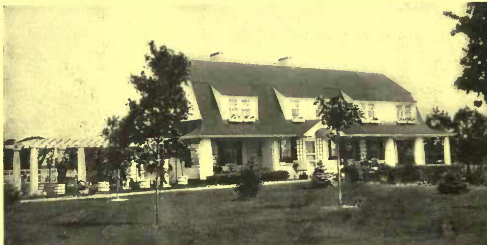
Porch columns supporting the extended roof should be solidly built and have lines of strength rather than beauty. I. H. Green, architect
