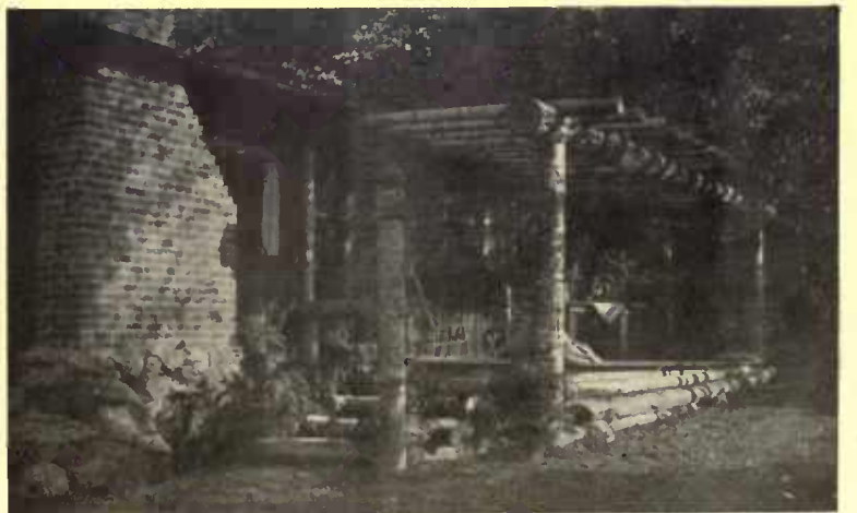
The pergola porch is in keeping with the rest of the house and has the advantage of being easily constructed
