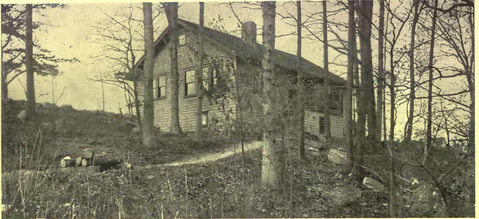
If the bungalow site is wisely chosen on a hill, it has the advantages of good drainage, a superior view and better ventilation
