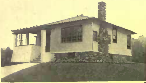
METAL LATH was used in this bungalow. Total cost ready for occupancy, only $2,400.
