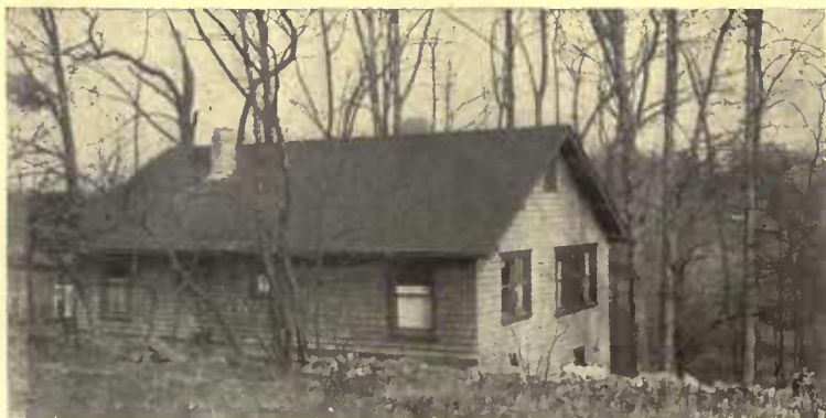
The original slope of the land was kept, thus avoiding the expense of cutting and filling, besides preserving a more attractive appearance
