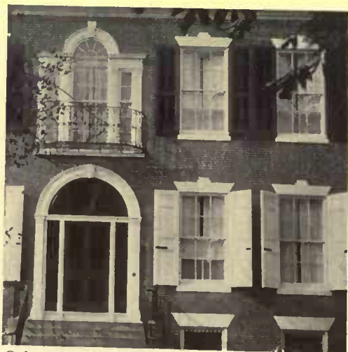
Colonial builders often used a Palladian window as the feature of the second story
