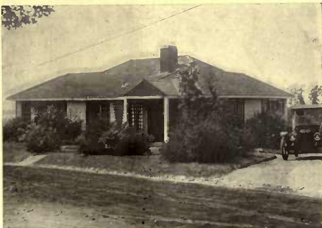
An unusual example of the value of strong horizontal lines in making the bungalow seem low and broad
