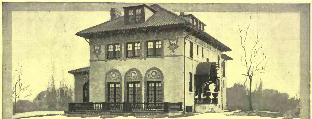
Residence of Mr. W. C. Calkins, Jr., at Flushing, Long Island. Frederick Squires, New York, Architect. A twelve room house exposed on three sides, with many casement windows, yet comfortably and economically heated with a Pierce-Spence Hot Water Boiler.
