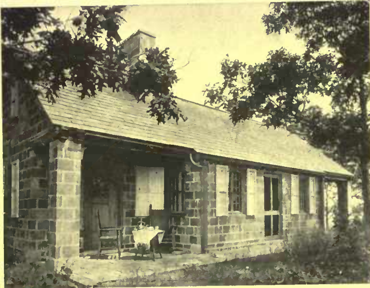
An interesting use of vitrified hollow tile that is particularly suited to small houses of the bungalow type
