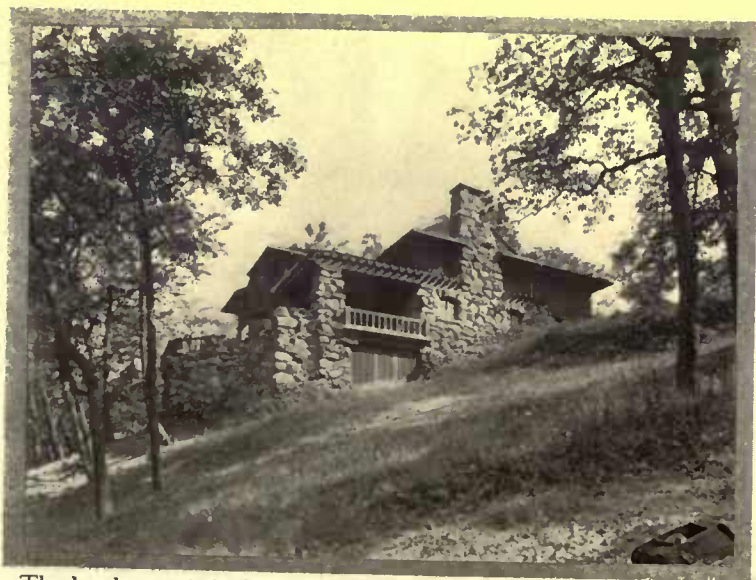
The local stone is built up to form a covered porch and terrace. The excavated slope saves in foundation cost
