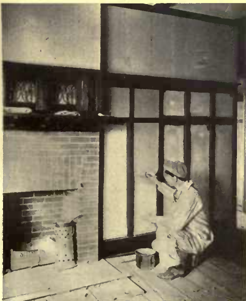
The various sorts of plaster or composition board are a reasonable and efficient substitute for plaster. They may be applied directly to the studing and if battens are used over the joints, successful approximate paneling is realized. They are ready for use and need only painting, but the directions for cutting should be carefully followed
