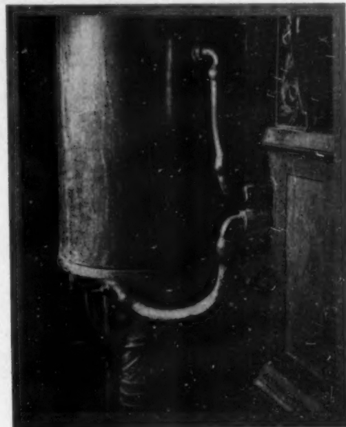
The lead pipe connections shown, although subjected to unusual strains from expansion and contraction, have lasted over twenty years and will probably last many more. Use lead connections
