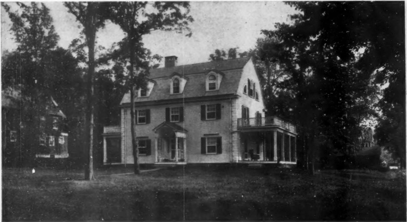
With all of the designers' conscientious following of precedent they have allowed themselves the luxury of two good porches in addition to the small entrance porch that alone was found on the old houses. The color scheme, of course, is white with dark bronze green blinds
