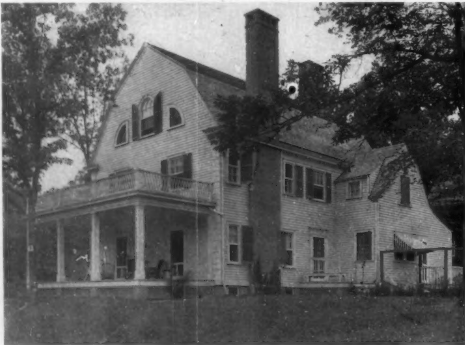
From the rear the house is as attractive as from the front, particularly in the sloping roof of the kitchen wing
