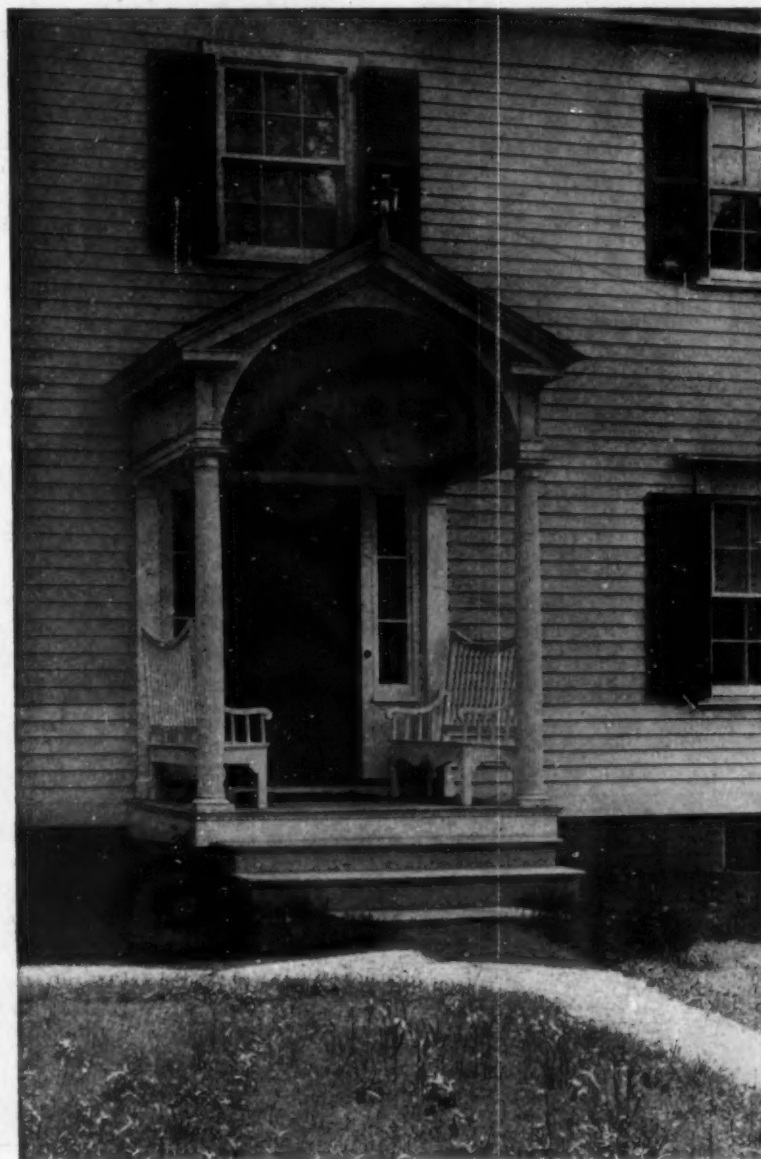
The entrance porch with its plastered ceiling is based upon an example on a Farmington, Conn., homestead
