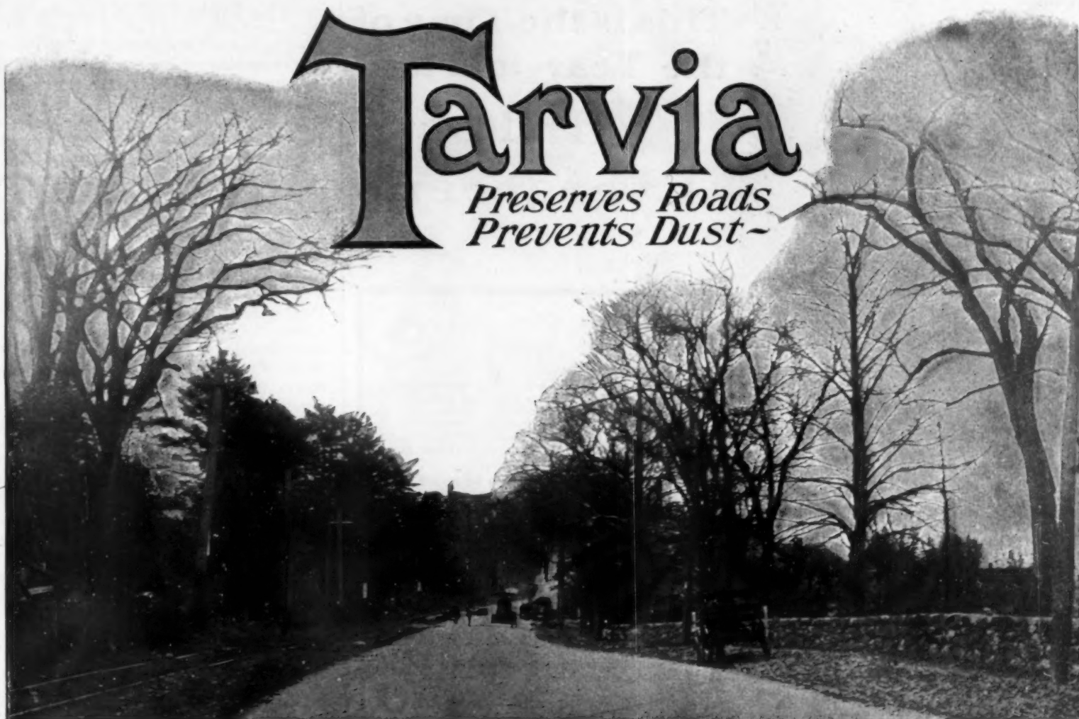
State Road, Watertown, Mass., Built With Tarvia X
