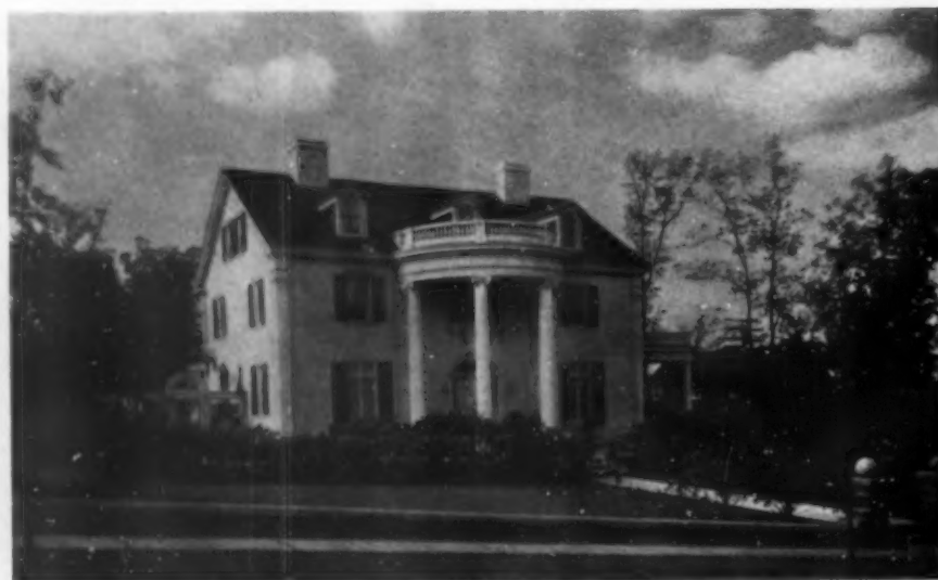
A typical suburban home where the service end is concealed by a well designed lattice reached from a branch path
