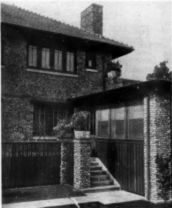
The veranda at the side of the house is screened and, as the first floor plan shows, is conveniently accessible from dining-room and butler's pantry
