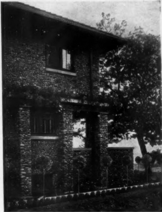
Looking along the side towards the front porch. The projecting piers carry the window-boxes
