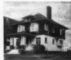
A No. 2-22-S IDEAL Boiler and 330 ft. of 38-in. AMERICAN Radiators, costing the owner $180, were used to Steam heat this cottage.
