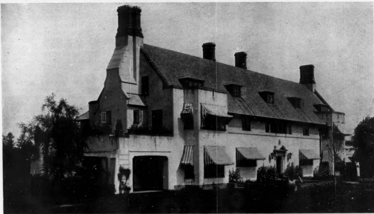
The home of Mr. Voorhees at Oak Lane, Philadelphia, where stucco has been used on metal lath in an English type of house
