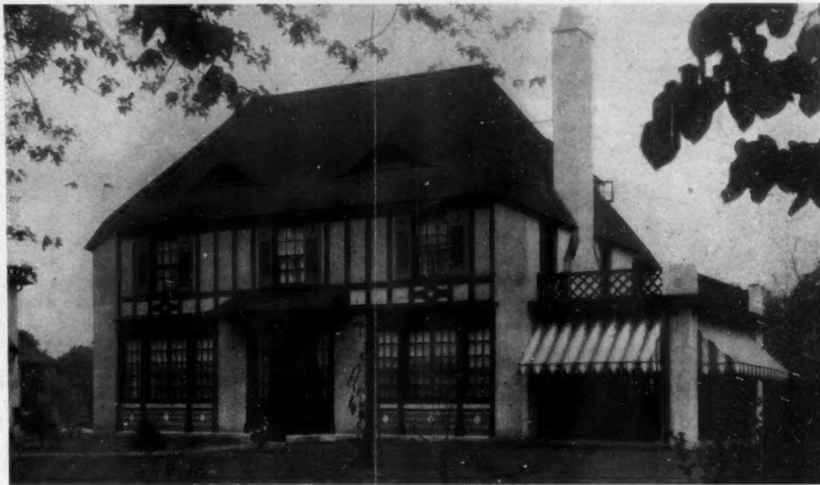
Stucco is perhaps seen at its best in conjunction with other materials, such as the half-timber work and the patterned brick screen wall in this house at Garden City. Aymar Embury, II, architect
