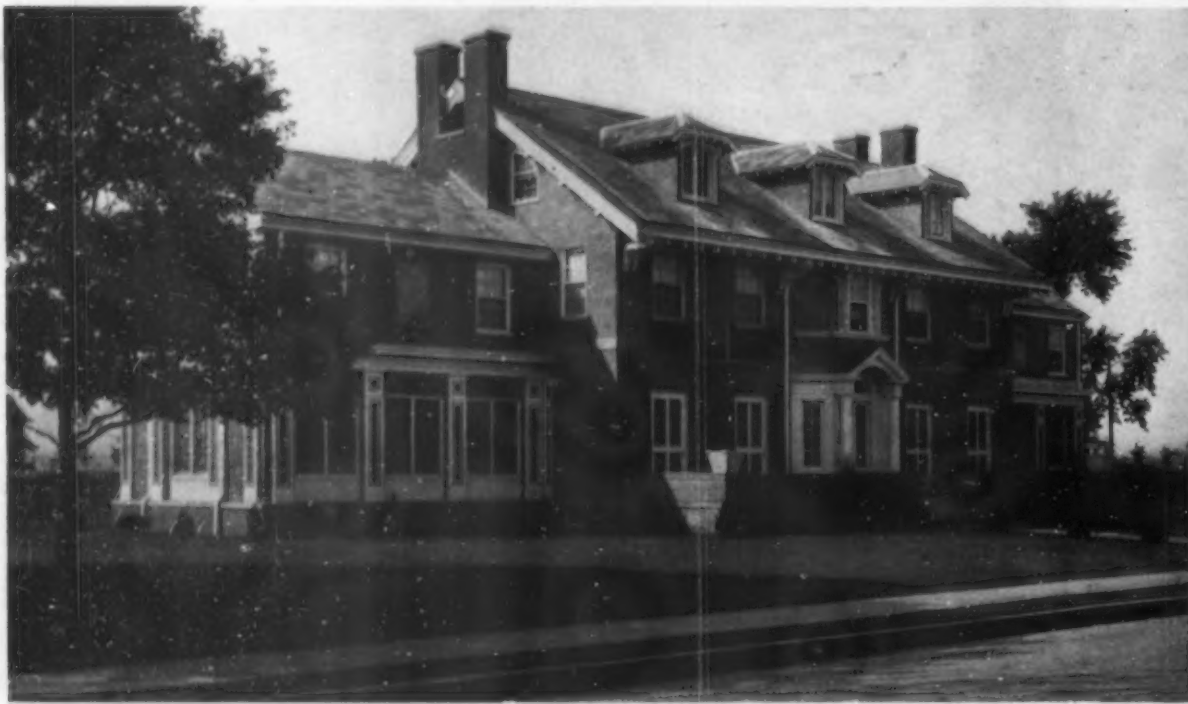
It is possible to secure dark stucco very easily, either by the use of colored aggregates or by the addition of mineral coloring matter
