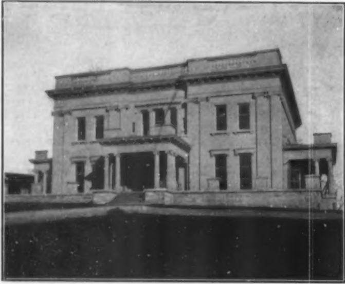
Residence of Hon. J. A. Howard, Wheeling, W. Va. Heated and Ventilated by the Kelsey Mechanical System
