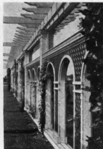
The green-painted lattice filling between the pergola arches relieves the white woodwork
