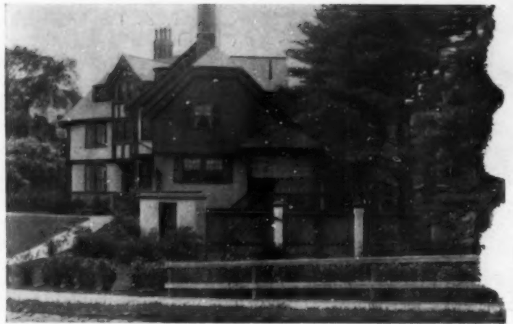
The laundry drying yard is well tied into the whole design by means of the extension wall and posts of stucco
