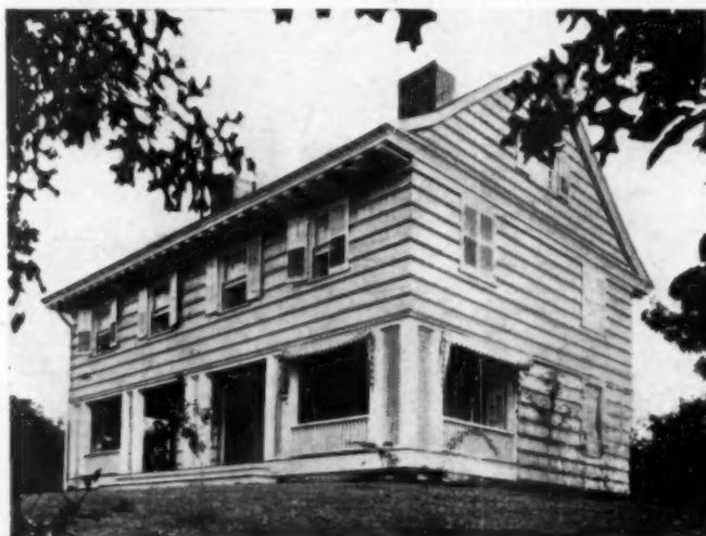
Latticework is effectively introduced to give more apparent strength to the supports in the home of A. W. Lord, architect
