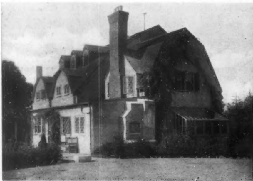
Most people, when thinking of greenhouses, picture only the large isolated ones that are expensive to build and heat. There is another kind, within the reach of every home-owner
