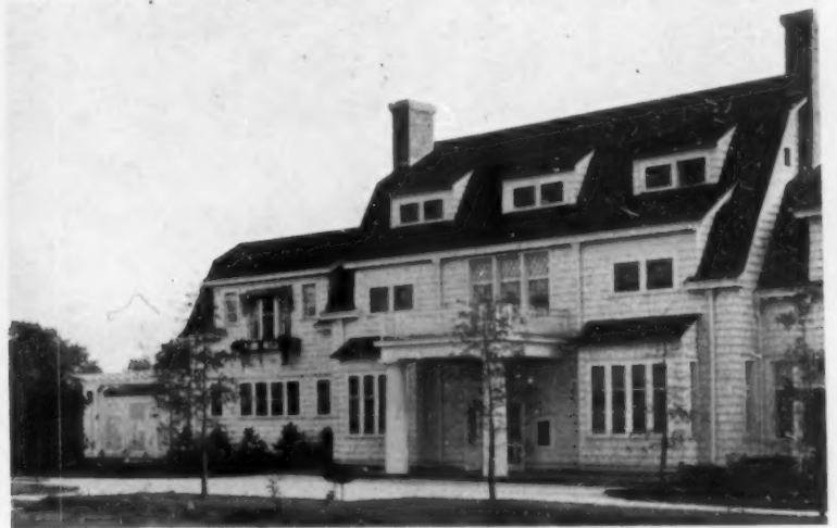
The lattice screen at the far end serves not only to conceal the clothes-line but increases the apparent length of the building
