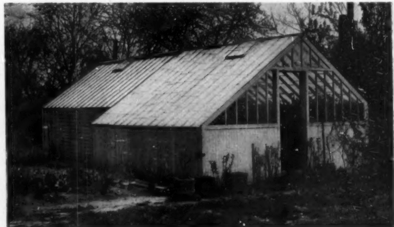
The home-made greenhouse of which the heating plant is shown above. It would be better to have a line of glass in the vertical walls just under the eaves
