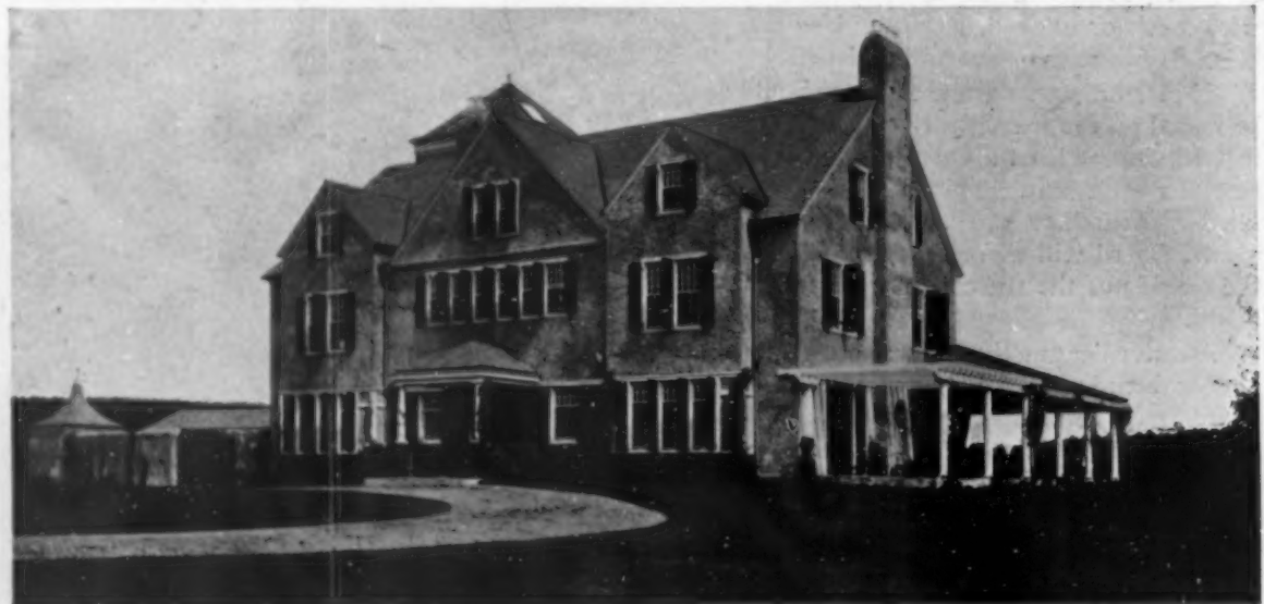
Particularly when stucco is used for the walls throughout is it advisable to secure in one of the many available ways a rough texture for the surface. "Renemedé," the home of Mr. H. J. Hardebergh, architect, Bernardville, N. J.
