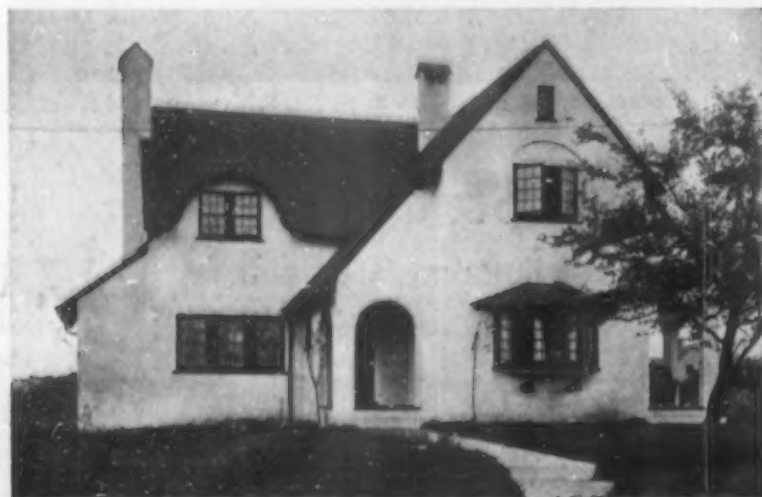
A house at Greenwich, Conn., that is of a type now being erected very widely in England with fairly smooth stucco walls
