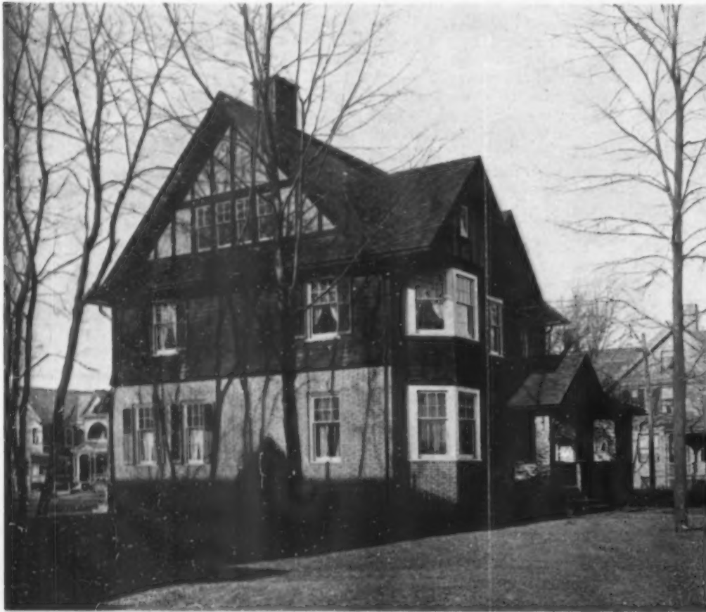
The Flemish-bond brickwork, dark stained shingles, the plaster-and-timber gable ends, and the white trim of the windows give a broad variety of materials that needs careful handling to be effective
