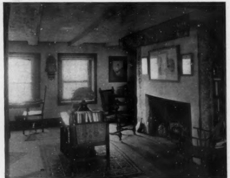
In the living-room the large fireplace has a plastered facing without any mantel. The old structural ceiling beams, painted white, remain
