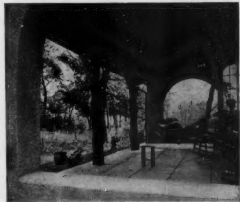
A covered veranda extends the whole length of one side, its roof supported by rough tree-trunk posts
