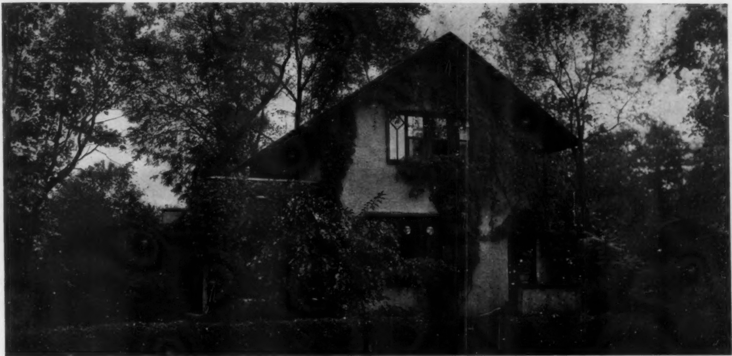
All plaster houses have a great advantage over wooden ones in that the walls need not be painted. The vine coverings need never be disturbed
