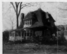
A No. C-241 IDEAL Boiler and 555 ft. of 39-in. AMERICAN Radiators, costing the owner $2260, were used to Hot-Water heat this cottage.
