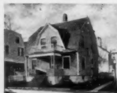
A No. 20 IDEAL Boiler and 240 ft. of 39-in. AMERICAN Radiators, costing the owner $1115, were used to Hot-Water heat this cottage.
