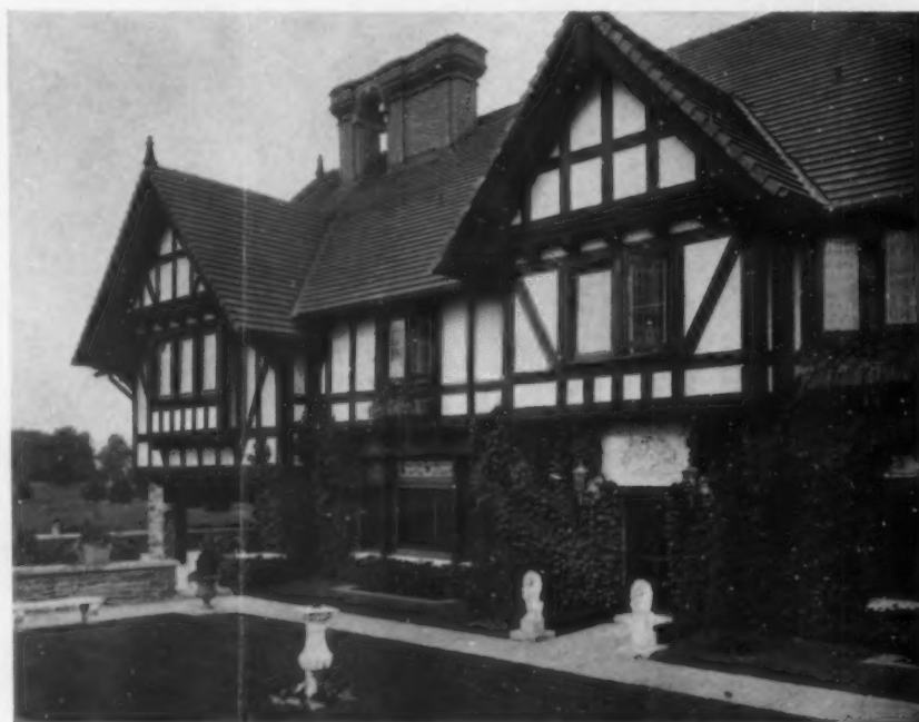
Unlike nearly all half-timber work in this country Lyndanwalt has been built with solid beams rather than the usual strip imitation
