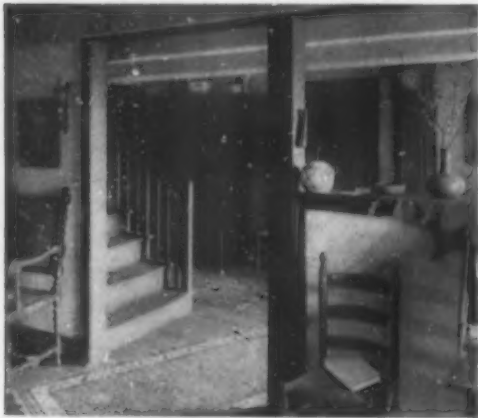
A view from the living-room into the central hall. At the right the partition is carried up only part way between the structural members, giving greater spaciousness to the interior
