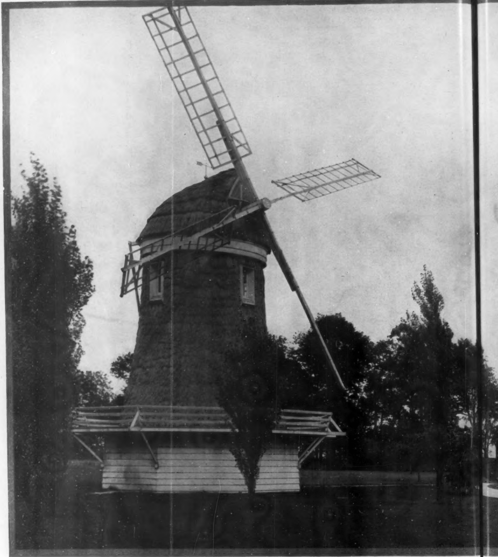
"LYNDANWALT," THE COUNTRY HOME OF MR. W. AT G The windmill is not merely a decorative feature of the estate; it actually supplies with
