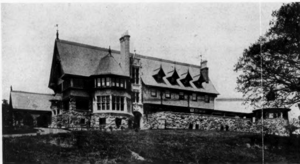
RESIDENCE OF E. J. LOBDELL, GREENWICH, CONN. Warmed by Hot Water System
