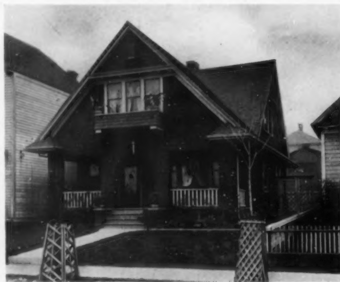
TYPICAL AMERICAN COTTAGE IN SEATTLE Warmed by water apparatus costing $250
