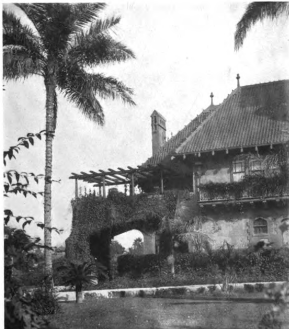
DRIVEWAY ENTRANCE COVERED WITH BOSTON IVY
