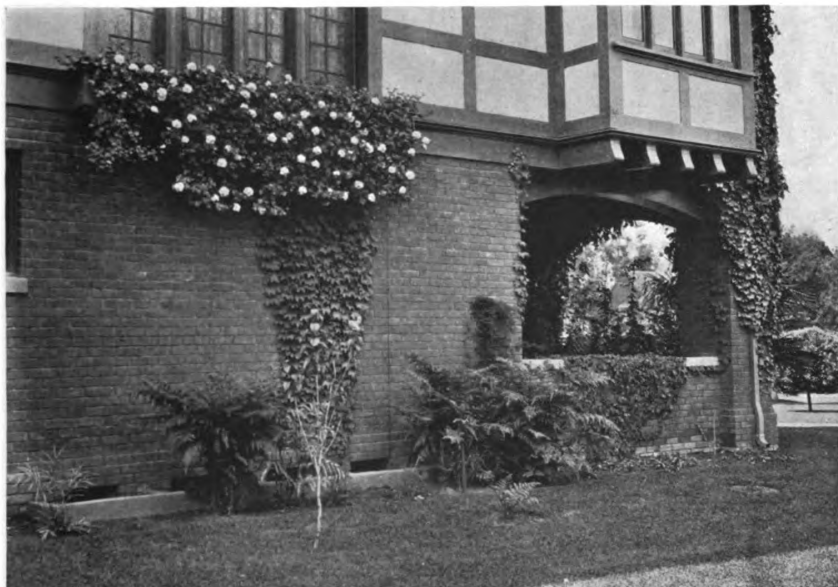
A WINDOW BOX AT WINDOW OF STAIRWAY LANDING
