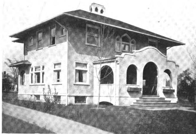
A Concrete Residence at Montclair, N. J. D. S. Van Antwerp, Architect
