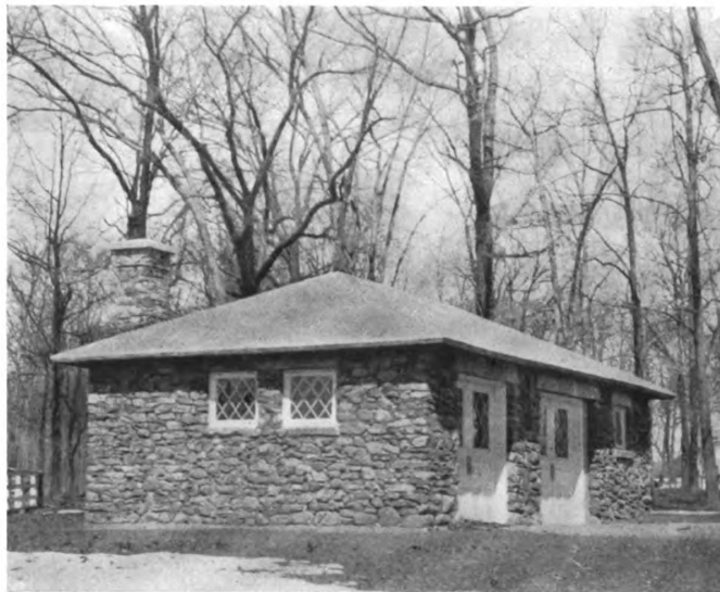
Garage built with walls of rough field stone backed with reinforced concrete and roof of reinforced concrete BENJAMIN A. HOWES, Engineer
