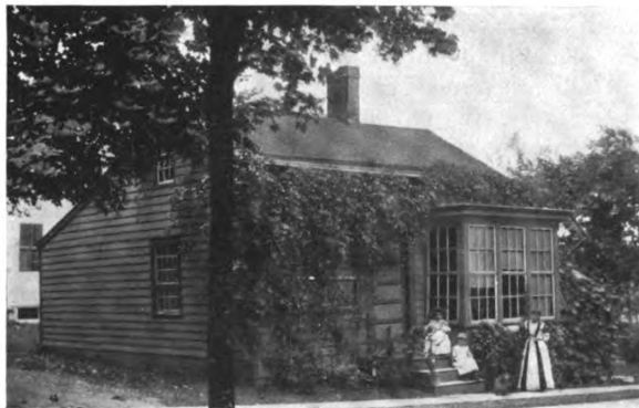
A cottage warmed by small hot water boiler and two radiators The boiler has a combination fire-pot, part of which is used to heat water for domestic purposes
