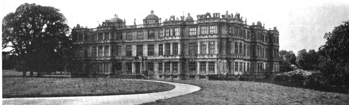
THE SOUTH FRONT OF THE HOUSE
