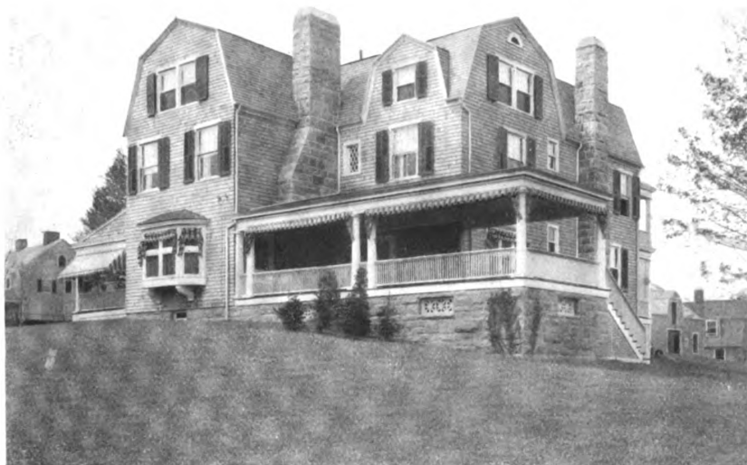
EXTERIOR VIEW OF "HILLSIDE"
