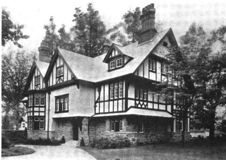
If proper equipment is installed, a healthy uniform temperature may be maintained with economy, in spite of wind and weather
