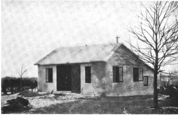
Garage built entirely of reinforced concrete BENJAMIN A. HOWES, Engineer
