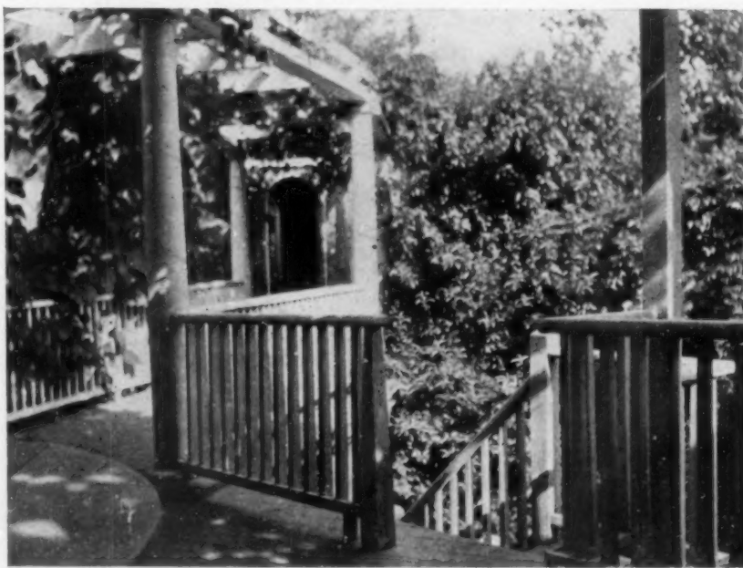
UPPER PERGOLA WITH ONE ENTRANCE TO ROOM IN TOWER
