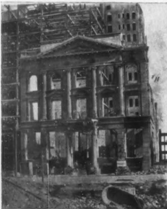
The San Francisco Gas and Electric Building. Stonework damaged. Brick and terra-cotta of upper stories undamaged though interior is completely gutted. The St. Francis Hotel in the background with steel frame of new portion unhurt
