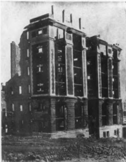
West Gate Apartments. Stonework completely ruined, enameled brick above, intact
