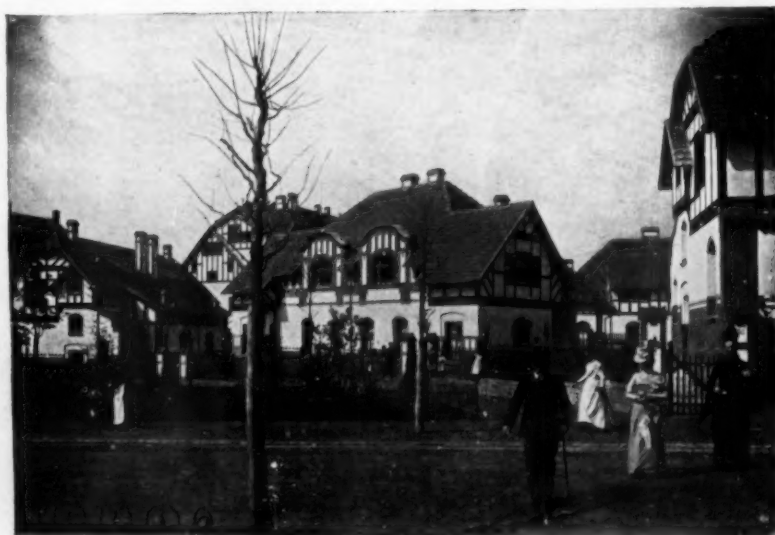
ENTRANCE TO THE COLONY FRIEDRICHSHOF SHOWING ONE OF THE TWO-FAMILY HOUSES ON THE LEFT
