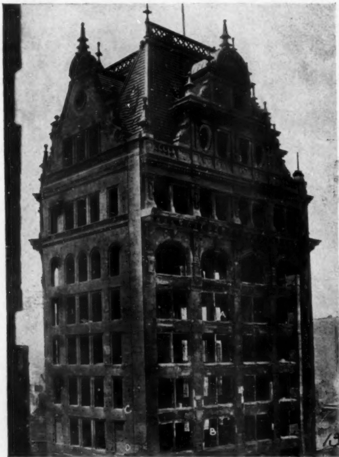
Mutual Savings Bank Building. The effect of fire on stonework. The terra-cotta gables were undamaged
