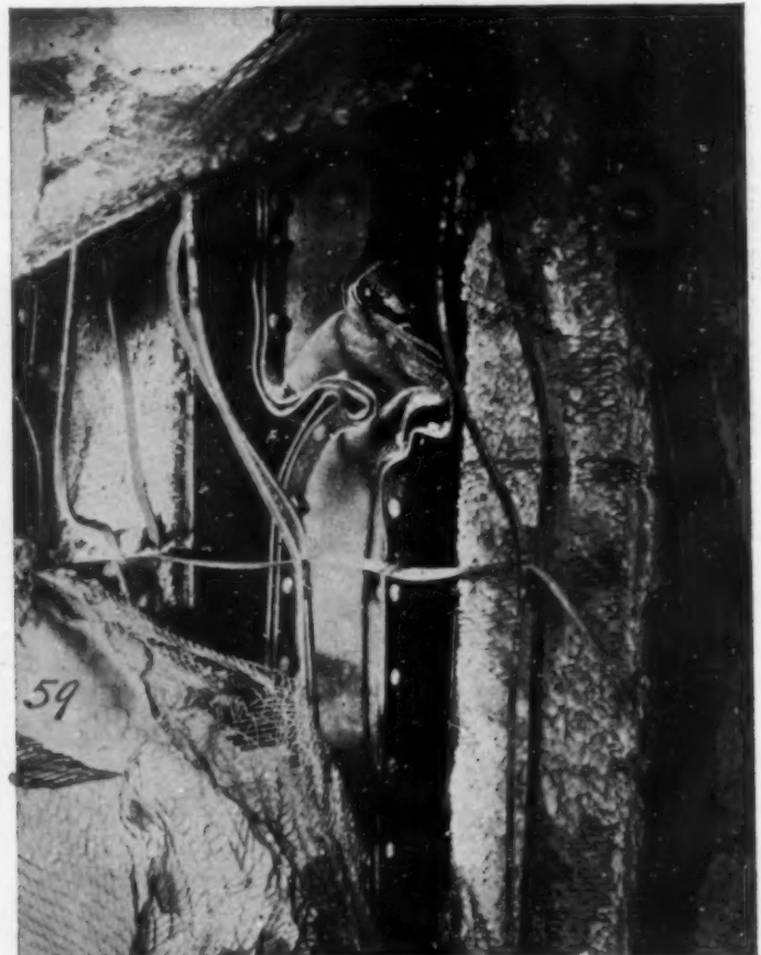
A column in the Fairmont Hotel, one of the newest buildings in San Francisco. Built under direction of leading architects there and alleged to be a model of concrete fire-proofing. It contained no furniture, nothing to burn except the floors and doors, yet it was damaged fully 50 per cent of its cost
