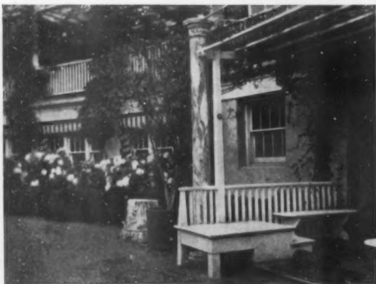
FRONT ENTRANCE, FLANKED WITH COLUMNS AND MOUNTING BLOCK
