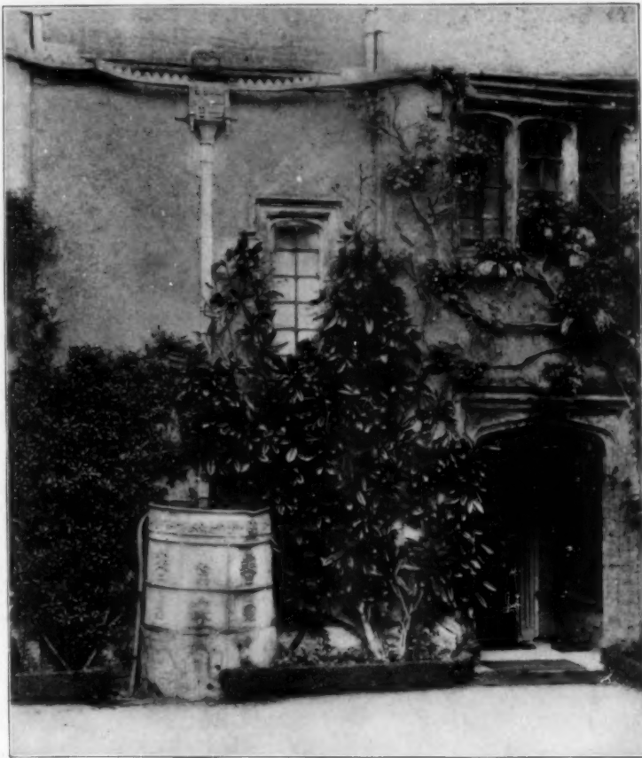
ARCHITECTURAL LEADWORK AT POUNDISFORD PARK
