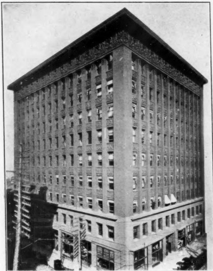
THE WAINWRIGHT BUILDING, ST. LOUIS
