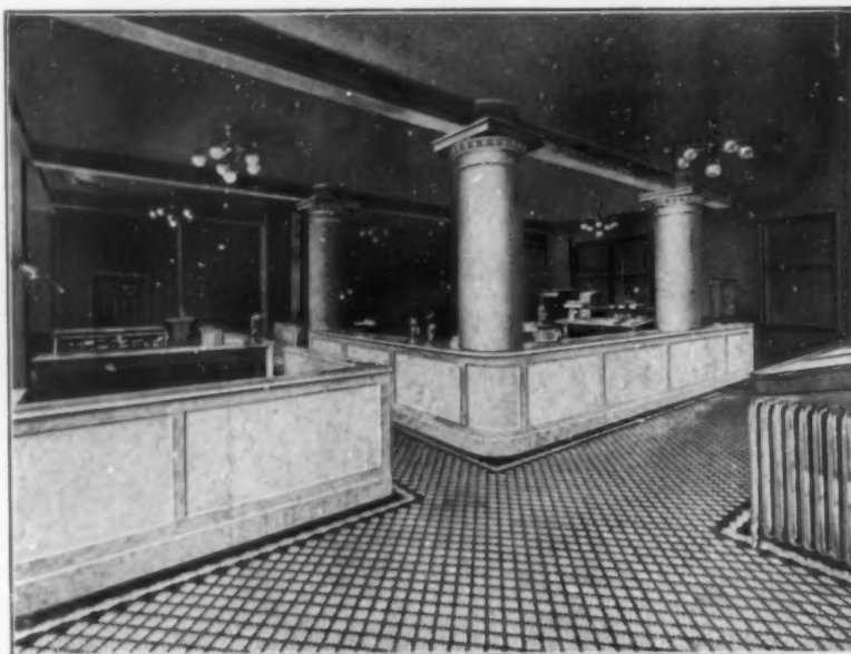
As laid by us in the St. Louis Star Building, St. Louis, Mo.
