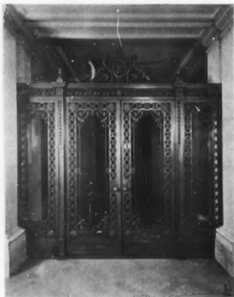
CAST BRONZE GRILLE DOORS IN MAIN CORRIDOR Second Floor Metropolitan Life Insurance Company Building N. Le Brun & Son, Architects
