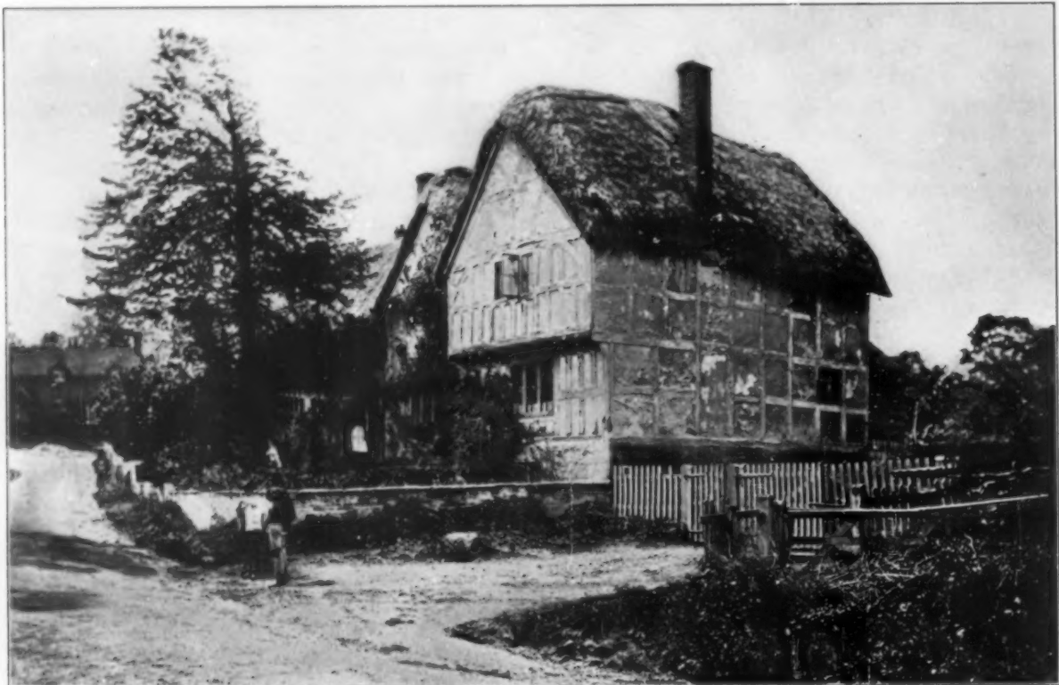
AN OLD HOUSE AT BRATTON
