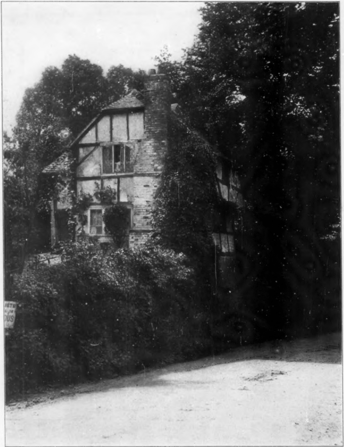
A ROADSIDE COTTAGE AT PULBOROUGH
