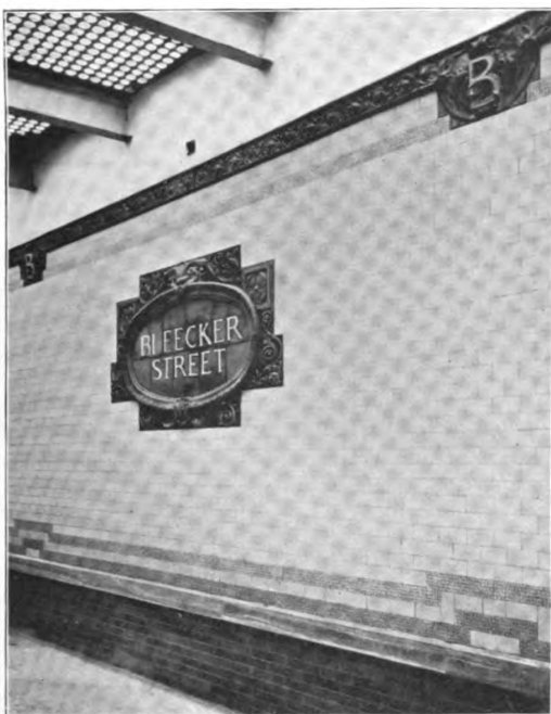
AT THE BLEECKER STREET STATION The ornament is of Grueby faience in a highly-glazed blue upon a white background
