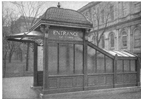
THE ENTRANCE TO THE SUBWAY AT CITY HALL Executed by the Hecla Iron Works
