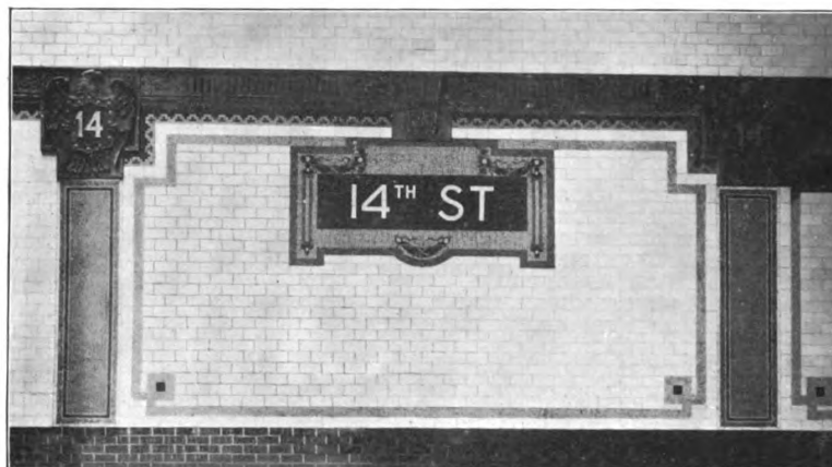
THE EAST WALL AT THE 14TH STREET STATION
