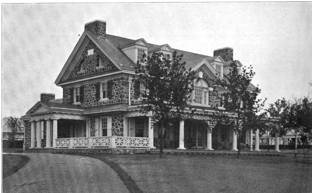
HOUSE OF PERCY WILSON, ESQ., AT DEVON, PA.
