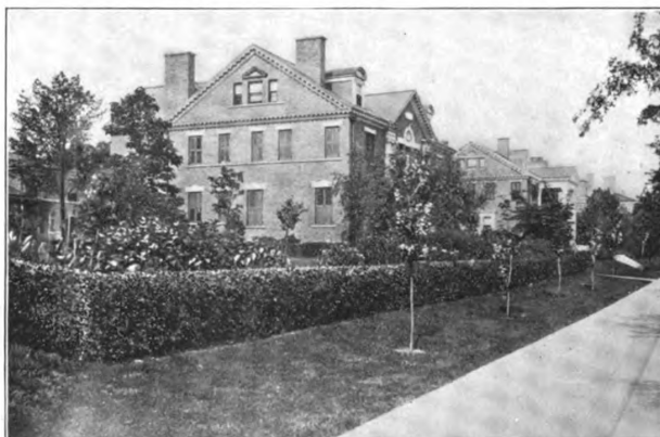
VIEW ON FOREST PARK TERRACE, WESTMORLAND PLACE Residences of B. B. Graham and R. S. Brookings, Esqrs. Eames & Young, Architects
