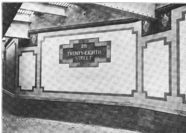
THE STATION AT TWENTY-EIGHTH STREET The Sign panel, cartouches and cornice are of Grueby faience in dull blue and buff, the letters being white. The walls are relieved by two shades of "glass tile" and mosaic
