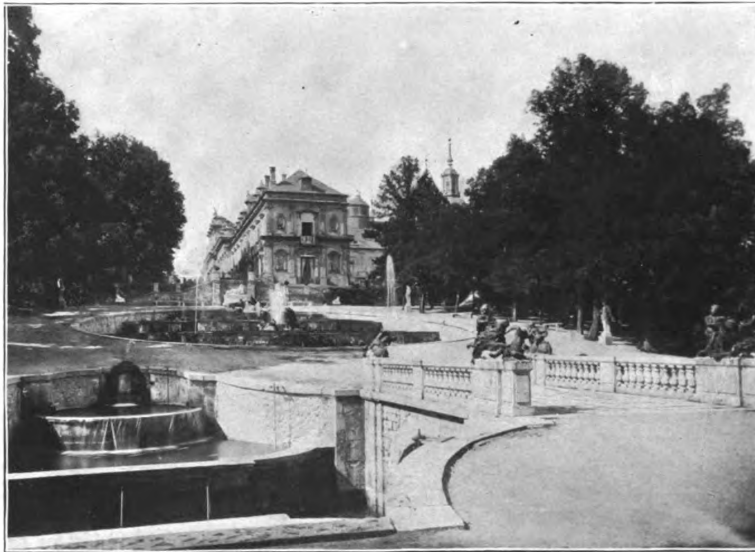
THE CASCADA DE LA SELVA AT SAN ILDEFONSO Illustrating a proper degree of landscape formality in the surroundings of a Palace
