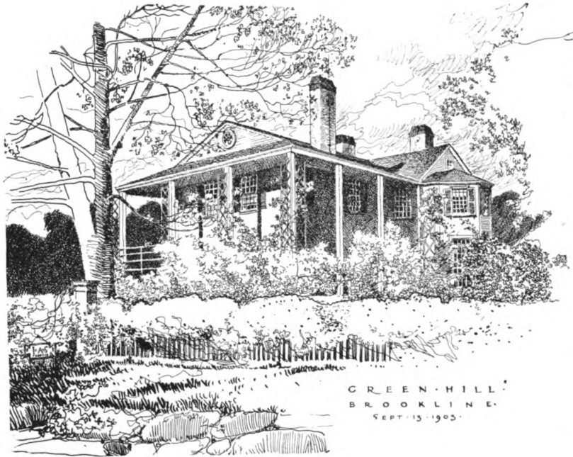
THE PILLARED VERANDA
