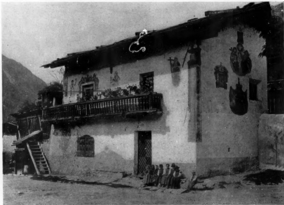
ON THE ROADSIDE AT LAATSCH
