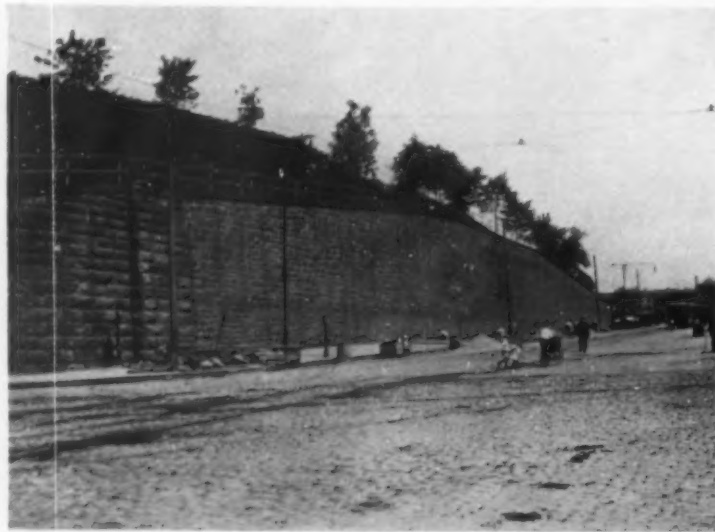
RESERVOIR WALL, PHILADELPHIA At the Green Street Entrance to Fairmount Park
