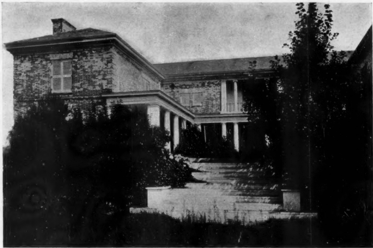
THE FRONT APPROACH, Photographed for HOUSE AND GARDEN in 1901 The Walls are of Red Brick Whitewashed
