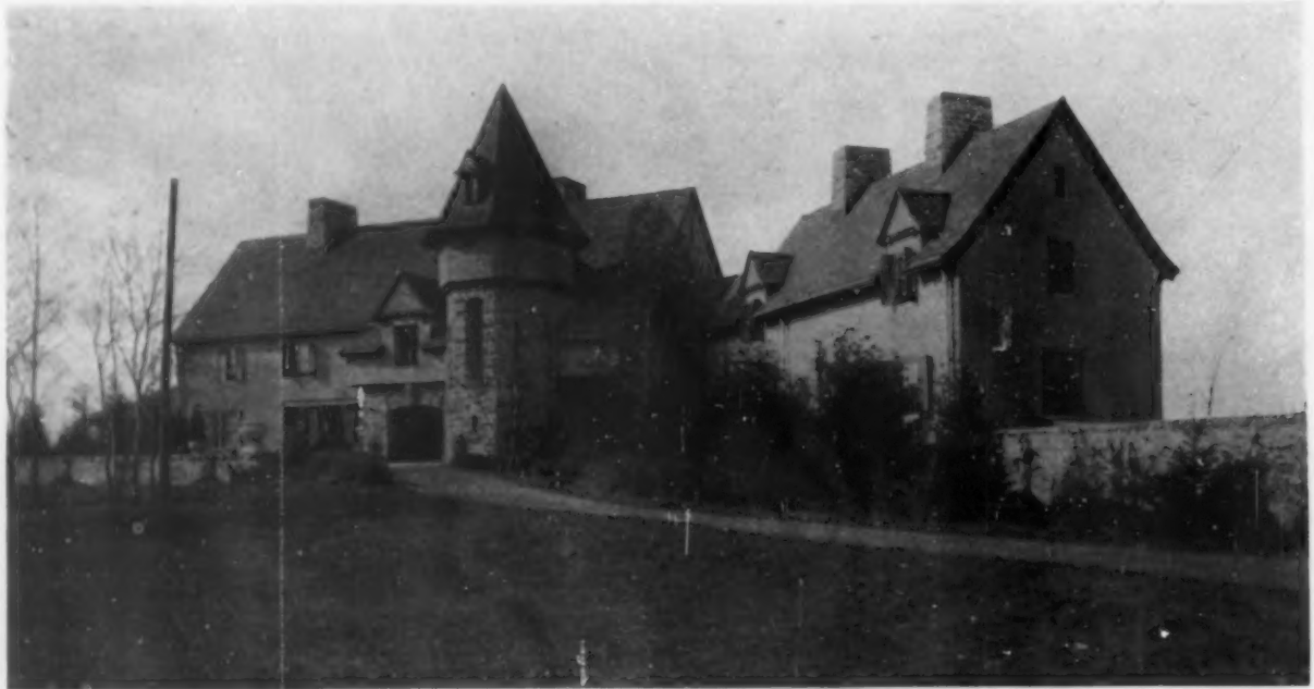
A HOUSE AT BERNARDSVILLE
