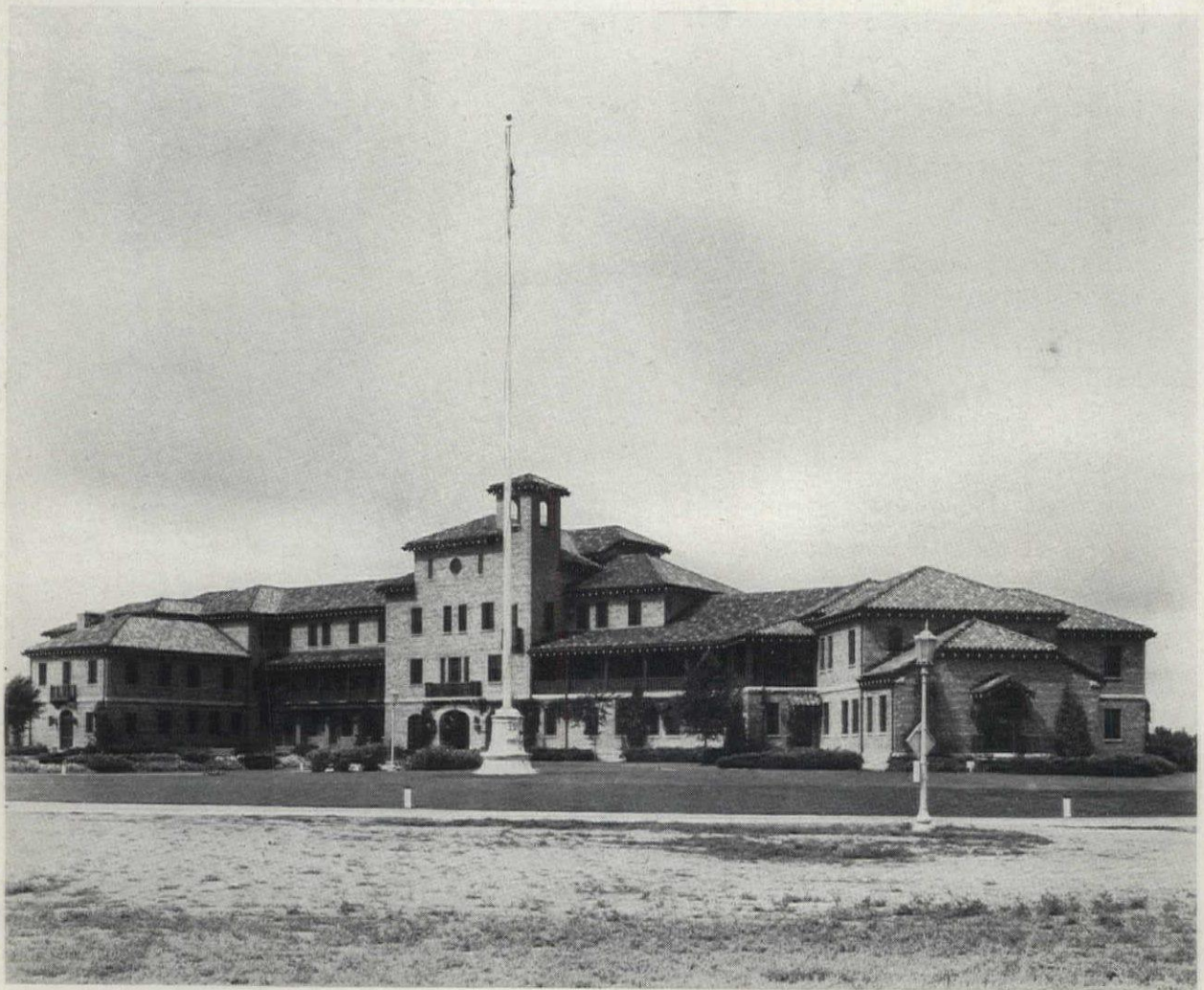
Main Hospital Building, Veterans' Administration, Cheyenne, Wyo.
