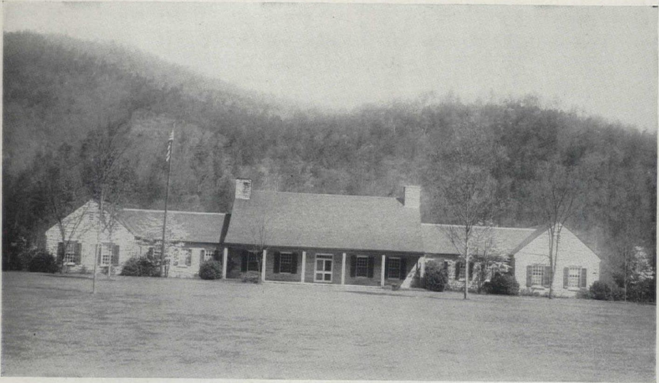
Administration Building, Great Smokies
