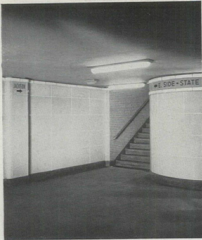
Glastone was selected for the walls of fifteen stations in the Chicago subway. More than 24,000 square feet of the glass faced masonry unit were used.
