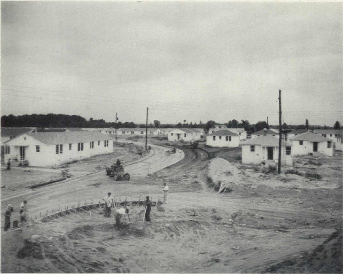
General view of the Bristol project.
