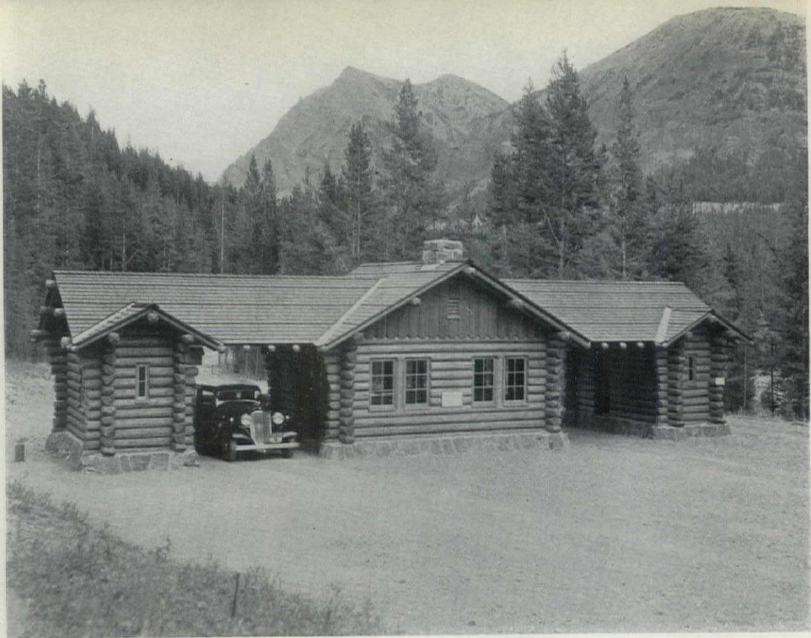
CHECKING STATION, COOKE ENTRANCE YELLOWSTONE NATIONAL PARK Branch of Plans and Design, National Park Service, Architects.
