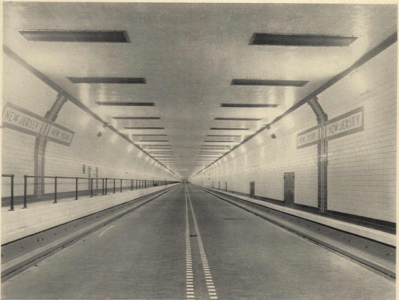
LINCOLN TUNNEL connecting Weehawken with 38th Street, Manhattan. Engineers . . . Port of New York Authority.
