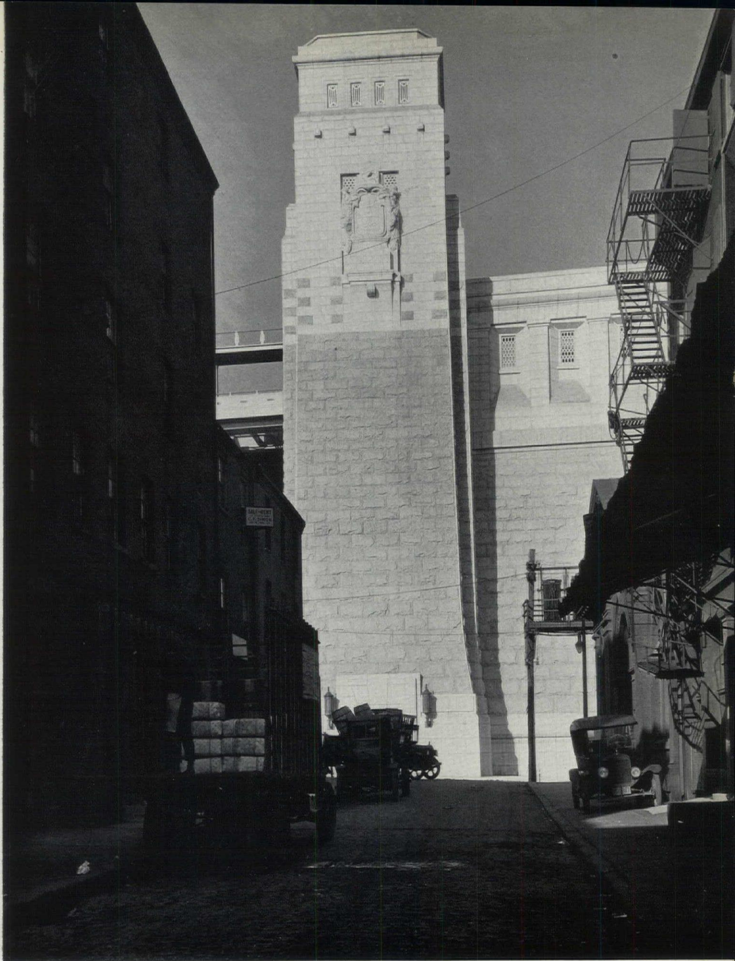
THE DELAWARE RIVER BRIDGE—ABUTMENT Architectural Design by Paul Cret
