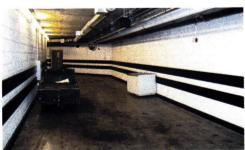
Durability of back-of-house areas often depends on the use of protective products, such as rigid sheet applied as a wainscot, horizontal quards, and door kick plates, all as shown here.
