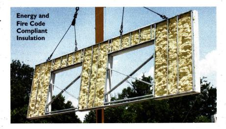
30 lbs. per sq. ft. composite panels containing 2 inches of precast concrete, are significantly lighter than traditional systems, allowing for larger panels and lower structural and foundation cost
