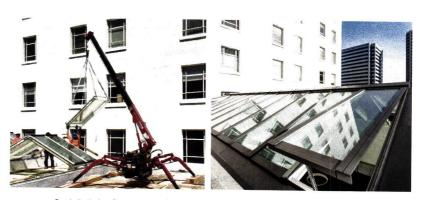
Due to limited rooftop space, a spider crane was used to maneuver the modular units into the ridgelight frames
