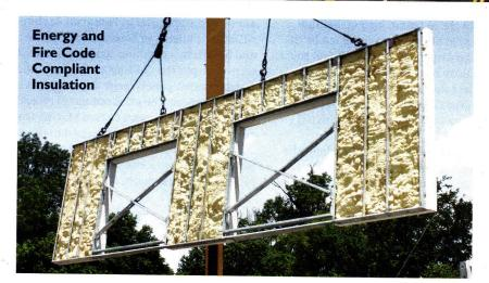
30 lbs. per sq. ft. composite panels, containing 2 inches of precast concrete, are significantly lighter than traditional systems, allowing for larger panels and lower structural and foundation costs
