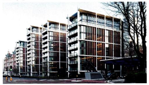
One Hyde Park, designed by Rogers Stirk Harbour + Partners, is tagged as 'the most luxurious address in London.' Crystalline concrete was selected for this project as a waterproofing and protection solution for the three-level basement slab and wall areas, attenuation tanks, podium slab, and penthouse roofs. It was also used for the traditionally cast and post-tensioned concrete, while also being utilized as a remedial solution for areas adjacent to the existing structure.
