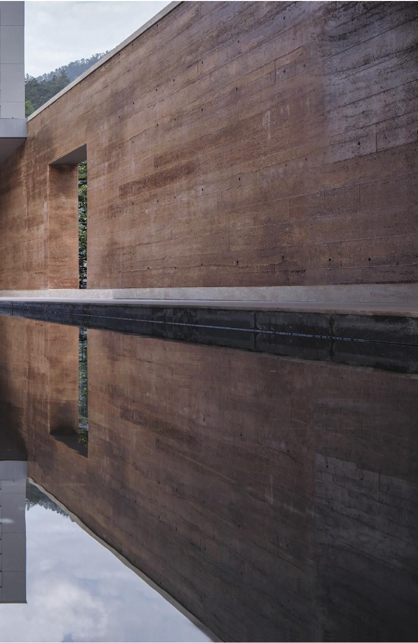
LONG AND LOW DL-Atelier conceived the San Bao Peng Art Museum (above and left) near Jingdezhen, China, as a 300-foot-long by 27-foot-wide compound defined by rammed-earth perimeter walls. Galleries are enclosed within titanium-zinc-clad volumes.
