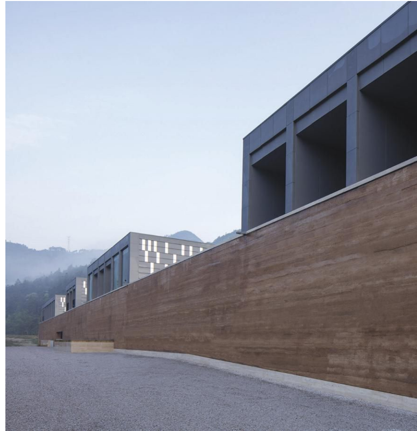
LONG AND LOW DL-Atelier conceived the San Bao Peng Art Museum (above and left) near Jingdezhen, China, as a 300-foot-long by 27-foot-wide compound defined by rammed-earth perimeter walls. Galleries are enclosed within titanium-zinc-clad volumes.
