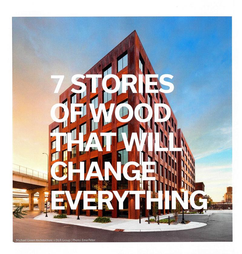
THINK WOOD T3 is a 7-story mass timber commercial building in Minneapolis that is signaling disruption in commercial development. Constructed with prefabricated NLT panels and glulam beams + columns throughout, it did not require code exemptions.
