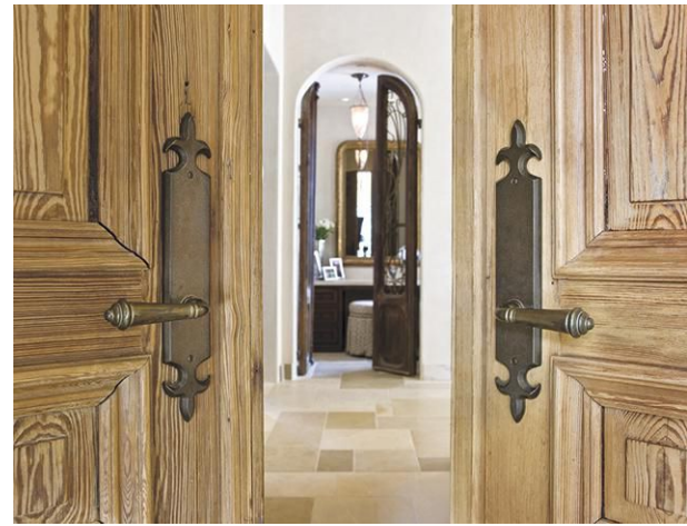
Classic Fleur de Lis hardware in silicon bronze medium was used for these reclaimed oak doors.
