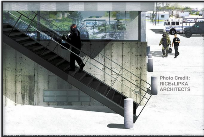
4x2 Multi-frame Smart Vent configuration installed on Bronx Bomb Squad building
