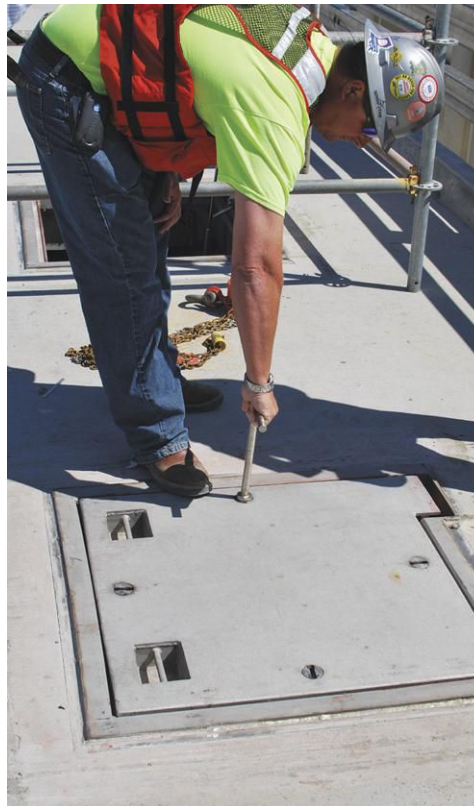
Rigid flood protection can include permanent or removable flood barriers, doors, and hatches that seal tightly against water and air penetration to protect people, equipment, and other valuables.
