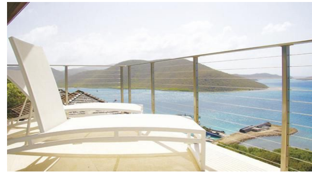
A stainless steel cable railing system provides panoramic views from this outdoor deck.
