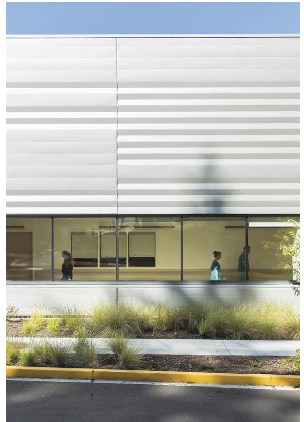
OF THE LAND The texture of the steel-panel cladding recalls glacial striations in the local landscape (above). Art and sculptural elements adorn the lobby (opposite, top), including decorative painted paddles, from the Tulalip Tribe, reclaimed boom logs, and reclaimed wood panels engraved with photos of historic Edmonds. Exam rooms surround the care-team stations (opposite, bottom).
