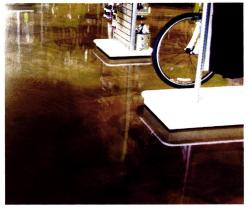
Resinous flooring, including polyaspartic coatings, provide a durable, attractive way to finish concrete surfaces.
