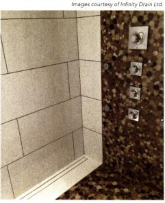
The design of shower areas in residential or commercial settings is streamlined by the use of complete shower systems that include waterproofed pitched floor substrates and tile backerboard as well as the decorative shower drain. The shower can be finished with tile or other materials, and the drain cover can be incorporated into the design as seen in the linear drain near the wall shown here.
