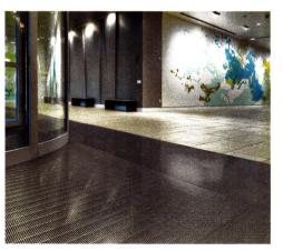
Entrance flooring systems can be incorporated into buildings to trap dirt, debris, and water from entering the rest of the building while being fully integrated into buildings, such as at Owego Elementary School in Owego, New York, (left) and the Westin Denver Airport in Denver (right).
