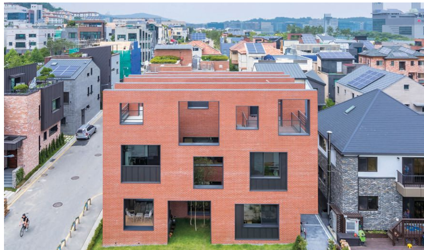
The Wall House features five 35-foot-high parallel brick walls (top). The perpendicular walls between them are clad in zinc (above). The distinctive design stands out among neighboring buildings in the low-rise residential community of Pangyo outside of Seoul (right).
