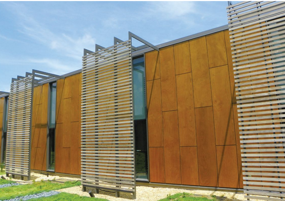
At the Owensboro Medical Health System in Owensboro, Kentucky, a natural wood rainscreen panel was designed to help support the image of a healthy, sustainable hospital.
