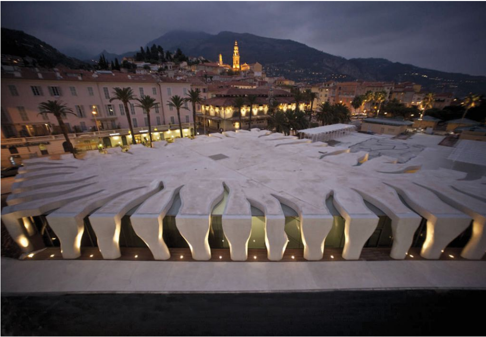
At the Musée Jean Cocteau – Collection Severin Wunderman in Menton, France, (2007), concrete is used to establish a rectilinear enclosure with a curved and flowing design expression.
