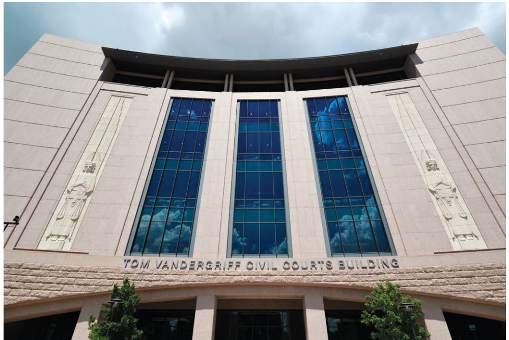
Tarrant County Civil Courthouse, Fort Worth, Texas
