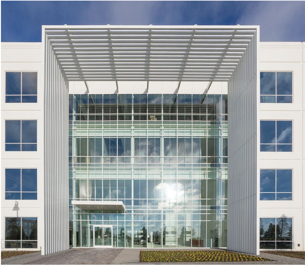
This GFF Architects-designed thermally broken curtain wall at the 9001 Cypress Waters office space in North Dallas, Texas, features unique T-shaped mullions and extended face caps.
