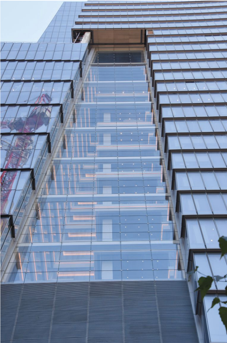
For the Kohn Pedersen Fox-designed 10 Hudson Yards in Manhattan, a point-supported structural glass system clads the 82-foot-tall cable wall lobby facade and a trapezoidal 207-foot-tall atrium cable wall for the 52-story high-rise.
