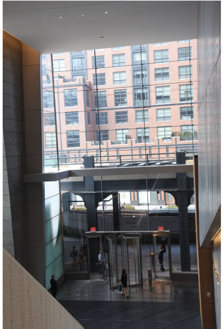
For the Kohn Pedersen Fox-designed 10 Hudson Yards in Manhattan, a point-supported structural glass system clads the 82-foot-tall cable wall lobby facade and a trapezoidal 207-foot-tall atrium cable wall for the 52-story high-rise.
