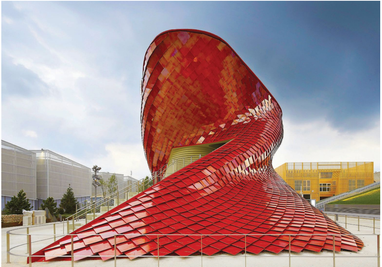
For Daniel Libeskind's Vanke Pavilion exhibition designed for the 2015 Milan Expo, invisible structural anchors were used to attach more than 4,200 tiles made from clay, quartz and feldspar within the free-form metallic facade.
