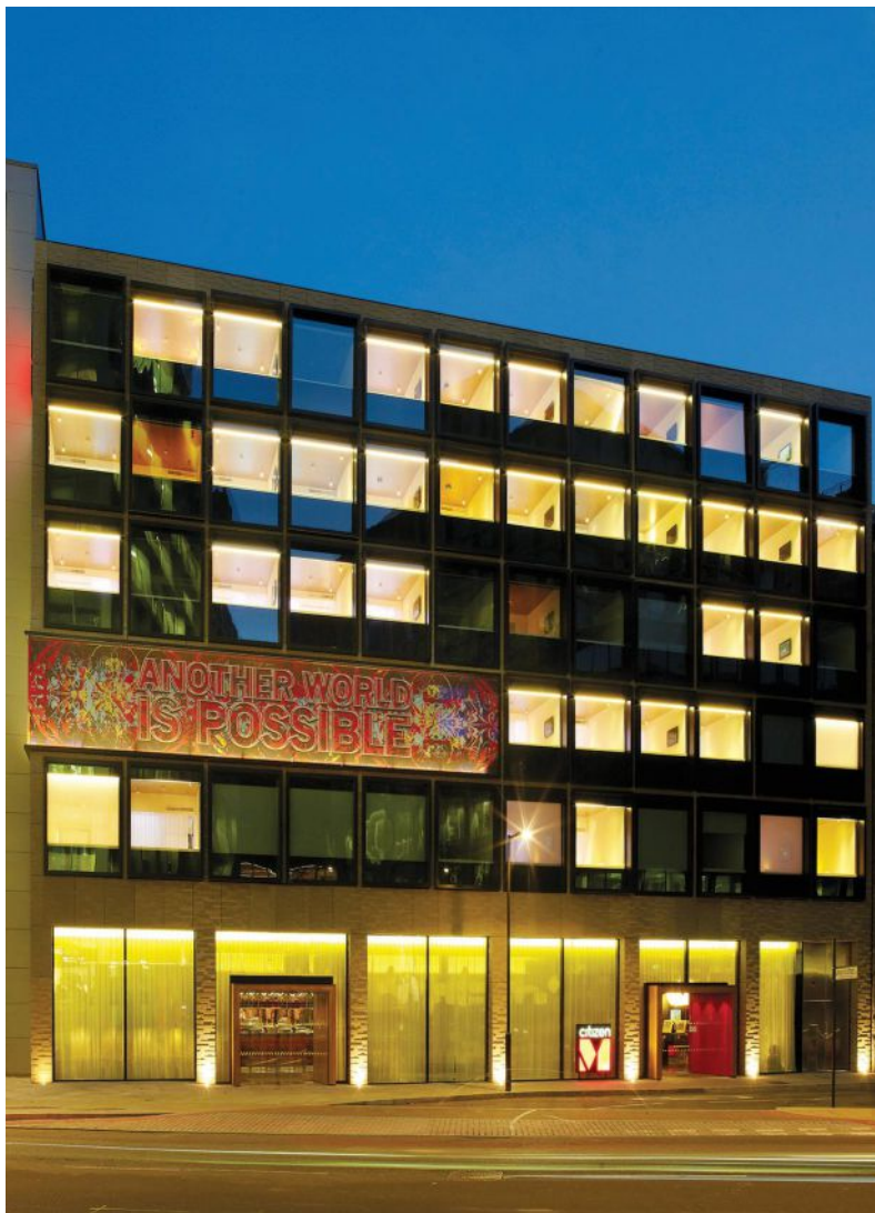
PACKING LIGHT The citizenM hospitality chain, which has nine hotels worldwide, including in London (left), constructs all guest room modules in Poland (opposite). The rooms, transported in shipping containers, arrive at the site with plumbing fixtures and furnishings installed (above).
