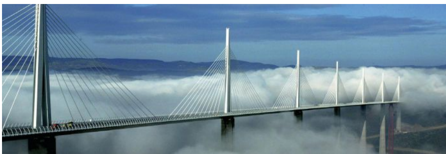
2004 Millau Viaduct Millau, France Foster + Partners
