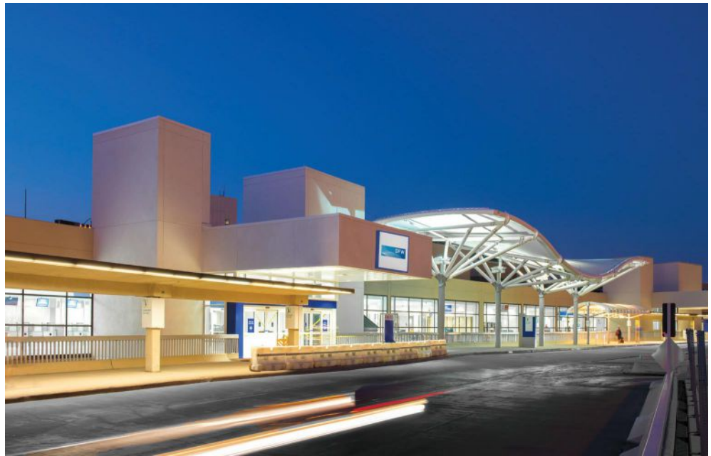
Limestone plaster was directly applied to new CMU and existing precast concrete along with frame/sheathing wall assemblies to achieve uniformity in texture and color at the Dallas Fort Worth International Airport (DFW).
