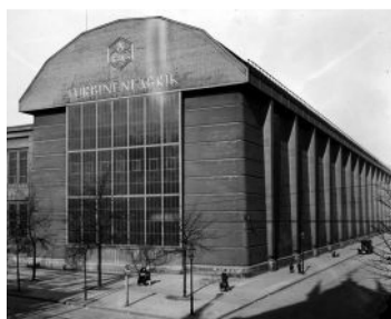
1910 AEG Turbine Factory Berlin Peter Behrens
