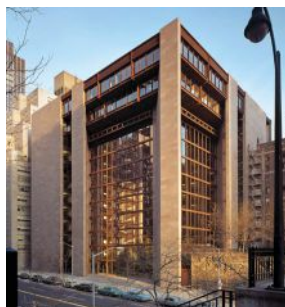
1967 Ford Foundation Building New York Kevin Roche John Dinkeloo & Associates
