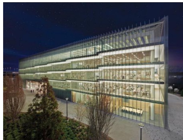
2013 Novartis Building 337 East Hanover, New Jersey Rafael Viñoly Architects
