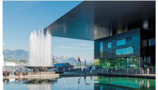
2000 KKL Luzern Lucerne, Switzerland Ateliers Jean Nouvel
