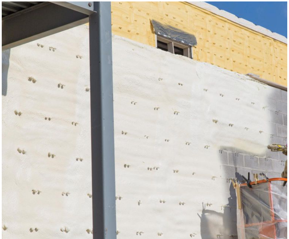
Medium-density, closed-cell spray foam insulation adheres to substrates and seals completely around cladding anchors, such as brick ties and other penetrations.
