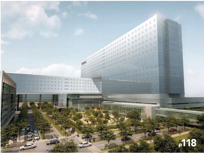
Image courtesy of Tremco Commercial Sealants & Waterproofing and BARA (Balfour Beatty Construction, Austin Commercial, H.J. Russell & Co., Azteca Enterprises)
