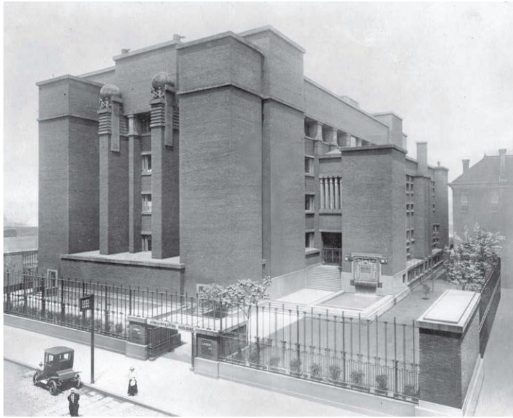
Wright designed a bi-nuclear plan, where the main building has offices arranged around a five-story light court, and the entrance and various services are in the adjoining annex.
