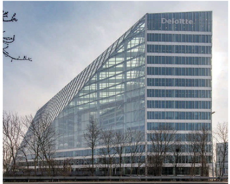
LIGHT MOTIFS The building's atrium faces north to benefit from indirect sun (above). Inside (opposite), the soaring volume shares its ample daylight with the surrounding glazed offices and elevator lobbies (which face it with fritted glass balconies).
