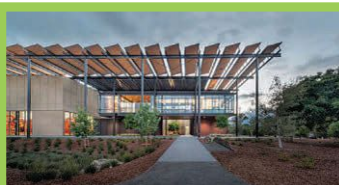
Stanford Energy Facility | ZGF | Stanford, CA
