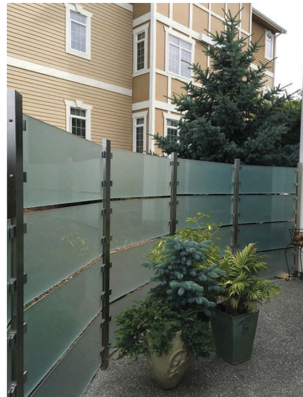
Glass as an infill material can help provide a sense of privacy, security, and also, when clear, open up visibility for occupants.
