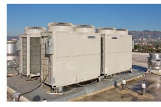
Variable refrigerant flow (VRF) zoning systems use centrally cooled or heated refrigerant run to individually zoned spaces based on the demand for space cooling or heating.
