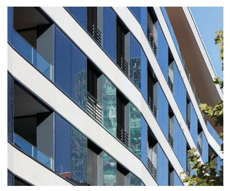
FACIAL TREATMENT In addition to the 770 conventional PV panels on the roof (below), Hegger Hegger Schleiff's apartment building in Frankfurt incorporates 348 BIPV panels into its facade (above). Together, the two systems generate a surplus of energy.
