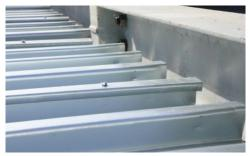
Composite floor metal deck systems can be designed with "upset" structural steel beams or with specially fabricated composite steel and concrete beams.
