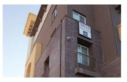
Architectural manufactured stone veneer can be used creatively in a variety of ways to enhance the texture and color of a multifamily building facade with quicker installation and less cost than conventional stone.
