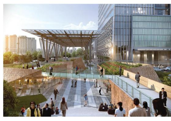
thin film solar modules embedded in the glass canopy. The challenge of the 80-foot-tall steelframe structure was to provide the retail and public areas with protection from the intense tropical sun and heavy rain while generating power, according to SOM's design development lead architect, Nicolas Medrano.
