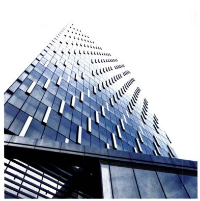
maintain comfortable indoor temperatures. In the winter, both poppers and floppers can be kept closed, allowing the air between the two skins to heat up and act as a thermal buffer, performing in much the same way as winter clothing. "It's like wearing a fleece with a shell over it," explains Benedict Tranel, a principal at Gensler and the project's technical director. "The inner facade is insulating, while the outer one keeps the water out."
