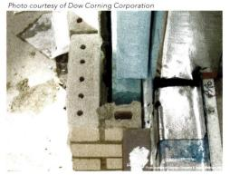
Self-adhered membrane installation at window opening—multiple layers and sequencing implications.
