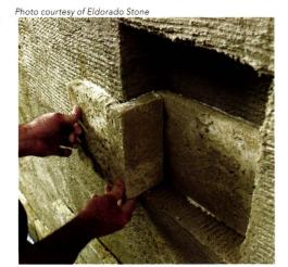
Wall transition using manufactured stone corner pieces.
