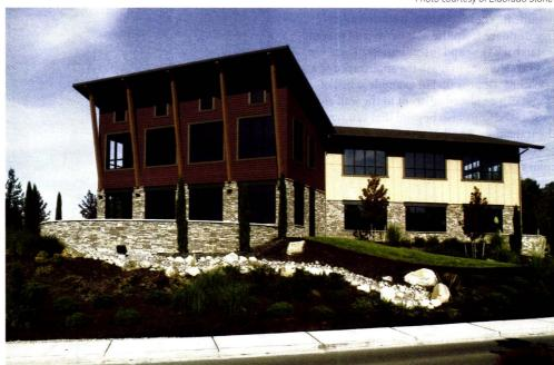
Installation of a manufactured stone system requires the choice of a believable color palette and careful placement of masonry units on exterior walls and building facades to maximize the illusion of natural stone.
