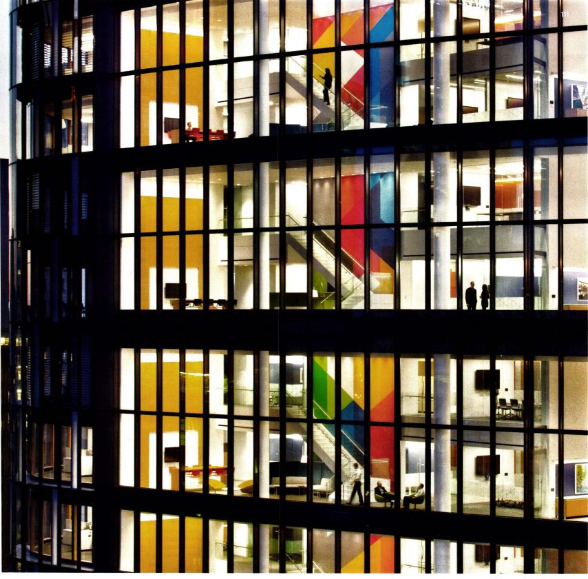
biggest contribution is the building's ability to "breathe." For a considerable portion of the year, the Tower at PNC Plaza will rely on operable windows and flaps in its sophisticated glass skin to bring in fresh air, rather than on mechanical ventilation. This move alone should produce significant savings, since the operation of HVAC systems is responsible for more than a third of overall
