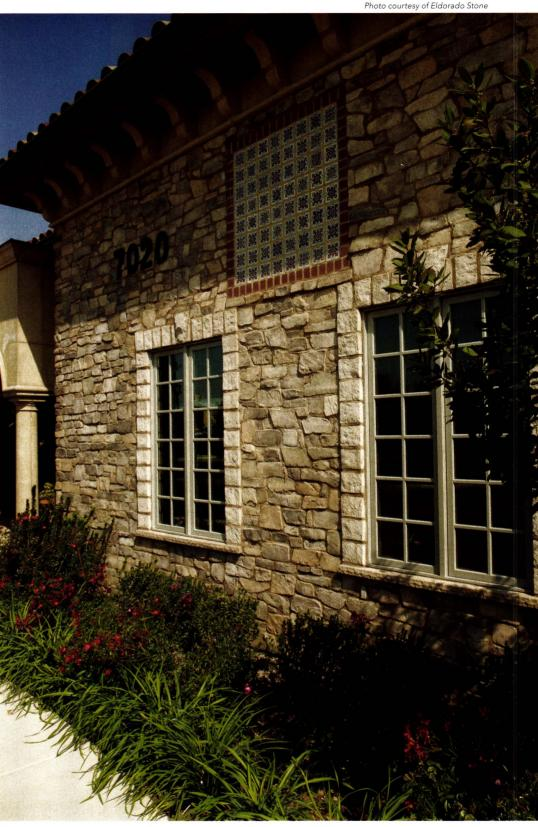
Foundation treatments that obscure the required termination of manufactured stone above grade can include a bed of stones placed adjacent to the wall along with a landscape area beyond that can screen the transition.
