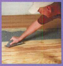
The underlayment features randomly air-laid filaments that create a capillary effect that cushions the floor and absorbs impact sound. It carries a Field IIC rating of 60 when tested under 3/8-inch glued-down engineered wood and when tested under ceramic tile, each time over 8-inch concrete with no ceiling assembly. The underlayment also helps smooth out imperfections in the subfloor and suppresses
