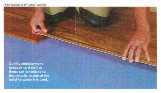
used, that material needs to be installed over something else. Hence, the choice of a suitable substrate with an appropriate underlayment material deserves proper attention. In the case of hard surface flooring in particular, such as wood or tile, the use of a performance-enhancing underlayment can help with design issues related to acoustics.
