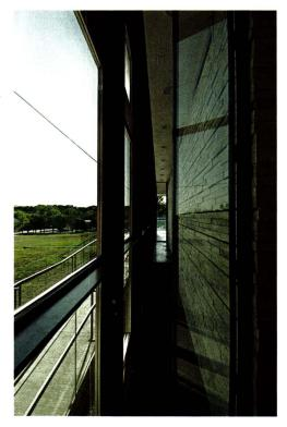
**CENTER FOR DESIGN RESEARCH** This LEED Platinum and Passive House-Certified project at the University of Kansas features a trombe wall behind an electrochromic butt-glazed curtain wall developed with SageGlass.
