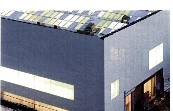
high, each one supporting the one above it and transferring dead loads to the foundation. The 140 panels were fabricated in Germany by Thiele Glas. German facade contractor MBM Konstruktionen coordinated their assembly at Thiele's factory, affixing aluminum supports to the back of the glass with structural silicone. These coat-hook-type elements fasten onto U-channels mounted on the building's exterior sheathing, facilitating installation.
