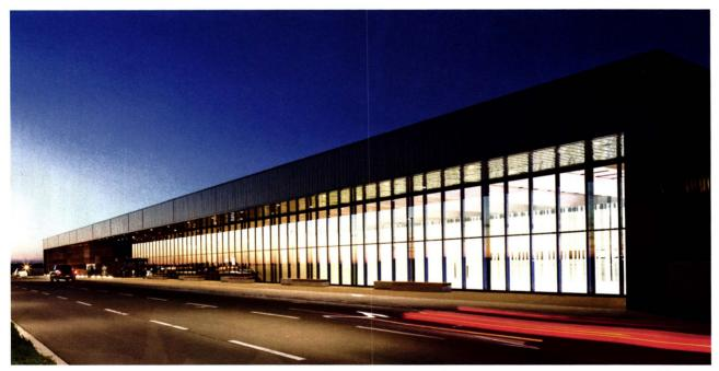
DRIVE BY The facade is defined by large Cor-Ten steel panels and a metal-alloy cladding that imbue the front elevation with a variegated texture (above). Most panel and window systems were prefabricated in southern Alberta to minimize on-site construction time. The departures roadway (left) is also the roof above the terminal's main entrance. The structure's floor-toceiling windows are triple glazed to contend with the region's minus-40degree winters.
