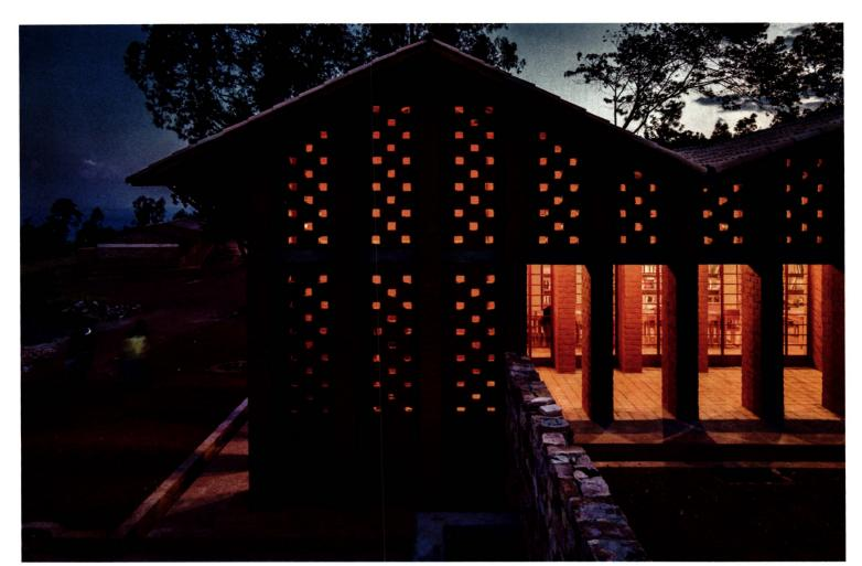
LOCAL HERO Using soil from the site for compressed-earth blocks, and local stones for mortarless walls helps anchor the 1,500-square-foot building to its physical and cultural context (opposite). Square spaces between the blocks aid natural ventilation in the library and the porch overlooking a courtyard (above). Wood shutters close the building when not in operation (right).
