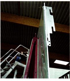
**OFF THE HOOK** The large glass panels were delivered to the site pre-assembled with coat-hook-like supports already affixed to their backs for easy installation.
