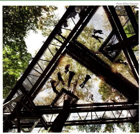
Galvanized steel was used for a human-sized bird's nest 80 feet above ground—and requiring no maintenance for more than 75 years.
