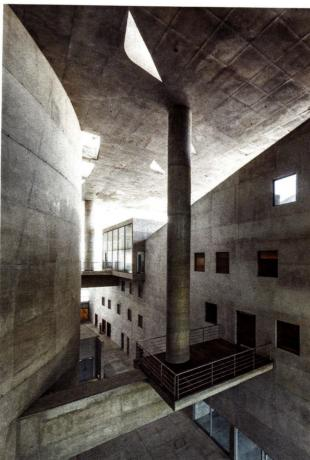
FLOTATION DEVICE Within the Cidade's single structural frame, separate volumes surround different components of the program, and flow open-air public spaces around them (above). Floating columns (left) distribute the weight of the roof to the enclosed spaces via transfer beams, one of which incorporates a small terrace on which musicians can have a break from the adjacent rehearsal room.
