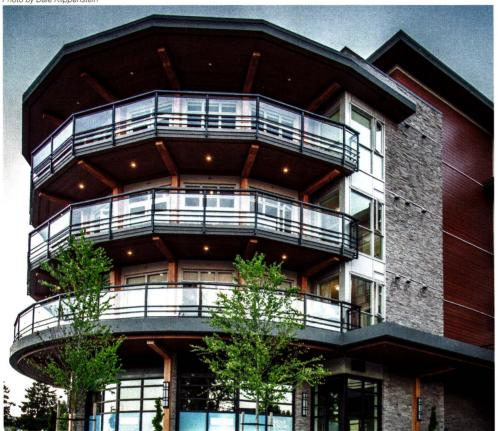
thermal bridge since there is often nothing to prevent heat from being transferred between the inside and the outside of the building along the entire perimeter of the floor construction. The obvious means to overcome this deficiency is to insulate this edge as part of the overall continuous insulation scheme of the building envelope.
