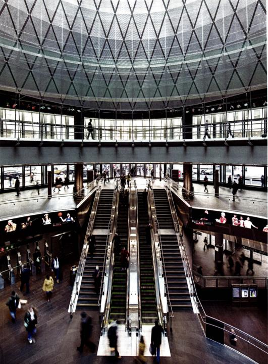
SUN CATCHER Fulton Center's key orientation element is the sky-reflector net, the product of a collaboration among James Carpenter, Grimshaw, and Arup. It consists of a skylight and 952 diamond-shaped perforated aluminum panels held in place by a doubly curved cable net. The device drives daylight into the station's lower levels and is activated by the sky's changing colors.
