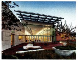
Recognized in the new IECC, integrated daylighting and dimming improves the efficiency of high-visibility façades as on the 367,000-square-foot, LEED Gold campus center for Gateway Community College in New Haven, Connecticut, designed by Perkins+Will.
