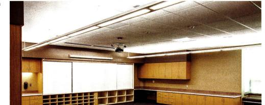
Recessed wall wash fixtures illuminate the white boards while indirect/direct luminaires provide general illumination at Sunset View Elementary School in Kennewick, Washington, designed by MMED Architecture.
