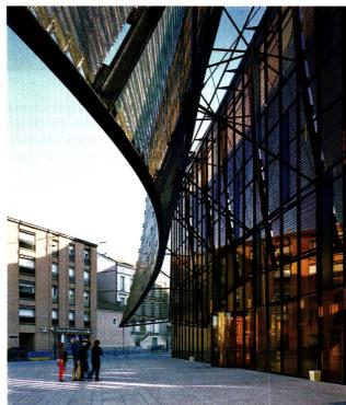
SCREEN PLAY Dominique Perrault Architecture wrapped the Albi Grand Theater in a metal mesh screen (left). It curves to catch sunlight at different angles and appears to change color throughout the day. The screen is attached to the boxlike building with a black steel armature (above).
