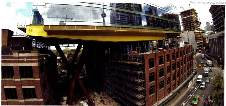
Architecturally exposed structural steel used on buildings of all types can now also be true design statements due to the availability of cast steel connectors in the U.S. and Canada.
