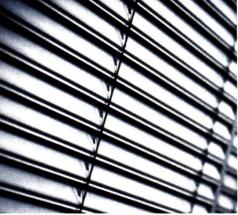
Conventional means of controlling daylight include vertical and horizontal louvers or baffles placed to re-direct and diffuse direct sunlight.
