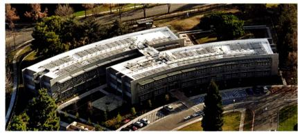
**EARTH STATION** Named in recognition of Tranquility Base, the first human outpost on the moon, the LEED Platinum Sustainability Base was designed to be an economic engine for built-environment technologies leading to independent, smart buildings. A pair of slender offset bars maximize daylight.
