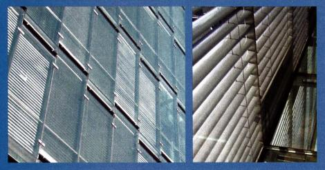
The Donnelly Centre at the University of Toronto incorporates perforated venetian blinds in a double façade on the south elevation. The blinds, in conjunction with the ventilated façade, provide effective solar control in both winter and summer months.
