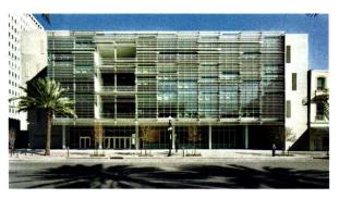
"wow" factor to do the job. The facade of the mostly glazed four-story structure features sunscreens to provide occupants comfortable levels of daylight. Interior amenities include a flexible 100-person conference center.
