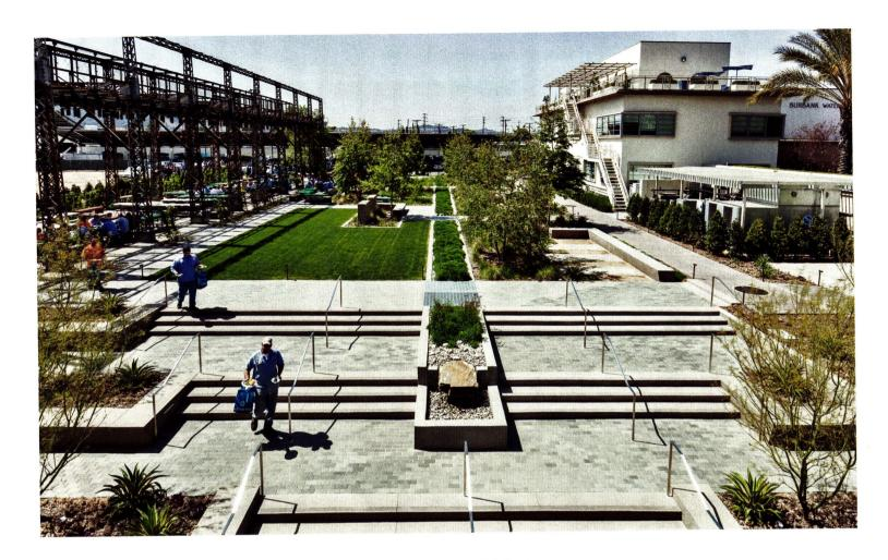
The centerpiece of the ecocampus stormwater management system is an old utility tunnel that designers converted into a filtration trench. The surface water and that of an adjacent building's green roof is fed into this trench, which is filled with gravel salvaged from the site and topped with plants that harmlessly absorb toxins from the runoff through a process called phytoextraction.
