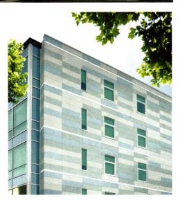
ABOVE: Fiber cement architectural wall panels are an advanced product compared to residential fiber cement siding and offer a full range of performance, aesthetic, and cost solutions.
