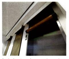
Smoke Guard manufactures code-compliant fire and smoke curtains designed to protect elevators, atria, and large openings with minimal design impact.
