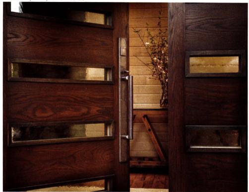
The increase in clean-line, modern hardware includes custom fabrication of building "touchpoints" such as handrails, door pulls, and other metal hardware in the high-end market segments. This residence has a high-quality door entry set in silicon bronze, with a dark luster finish.
