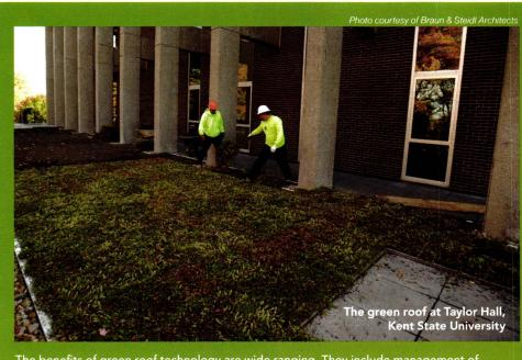
The benefits of green roof technology are wide ranging. They include management of stormwater, reduction of heat island effects, restoration of habitat, biodiversity of plant and wildlife, water efficiency, energy optimization through both cooling and heating, reuse of building materials, recycled-content materials, increased roof durability and longevity, and creation of rooftop amenity spaces.
