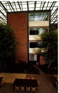
Fire-resistive glass vision systems are being utilized effectively to block flames, smoke, and radiant heat for up to 2 hours, in lieu of traditional opaque walls or glass block.
