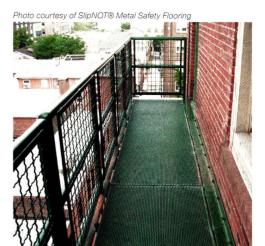
Architects specify slip-resistant metal floor components to eliminate hazards while still complying with ADA or OSHA requirements.
