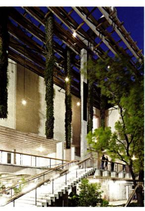
Thin concrete columns support a wood canopy hung with strands of vegetation.
