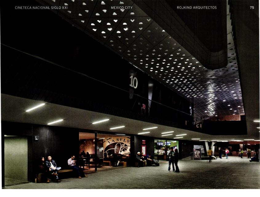
become a 120-foot-long canopy. The span connects the new building to the existing theaters and creates a sheltered plaza below. The dramatic steel construction is clad in composite aluminum panels perforated with triangular openings that widen and narrow to control the amount of sunlight passing through the covering.
