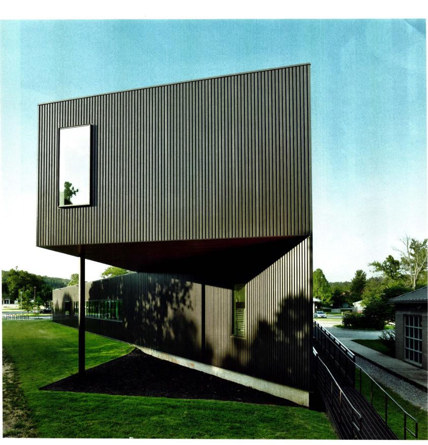
SHARP TAILORING To give workaday metal cladding a level of polish, the architects collaborated with fabricators to create custom cap pieces for the rear corner of the triangular first floor. The detail refines the building's geometry and adds a sense of seamlessness to the facade.
