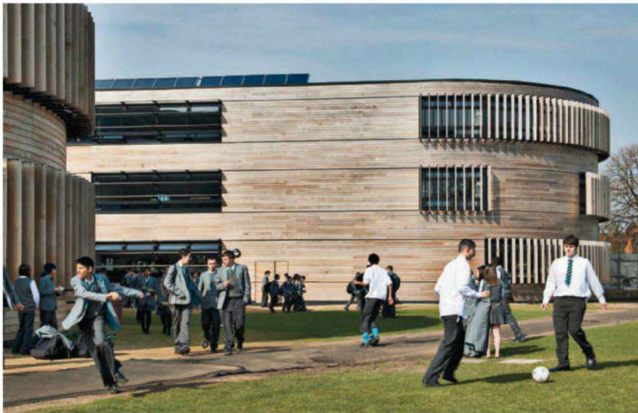
Foster + Partners' Langley Academy, with its curved facade, would not be sanctioned under new rules.
