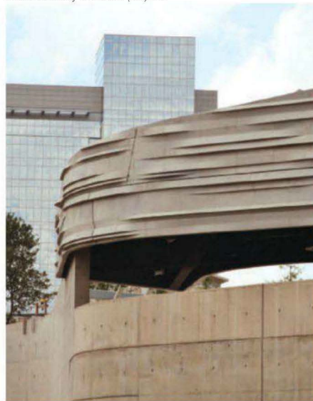
The concrete mixes for the project included up to 51 percent slag in core walls, and 50 percent fly ash in piers, columns, and slabs.
