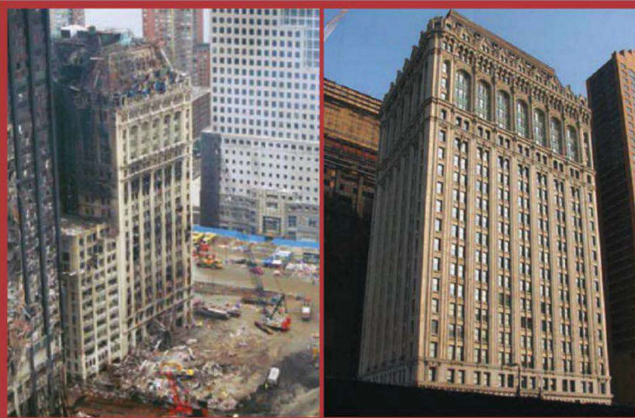
Demonstrating the resilience of CMU, the West Street Building by Cass Gilbert was reopened in 2005 after being damaged by the World Trade Center collapse and a five-day fire in 2001.
