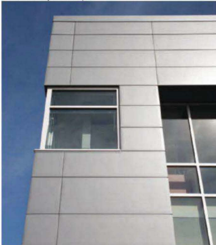
An insulated metal panel system at Pacific Plaza, Tacoma, Washington, provides an air and vapor barrier. Architect: BLRB Architects.
