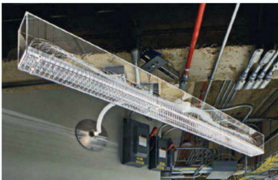
LIGHT PIPES Linde has custom-designed fiber-optic lighting fixtures (left) that guide sunlight from the coelostat into the laboratories. The illumination system includes silvered mirrors and lenses housed within optical tubes (above) for concentrating and directing the daylight.
