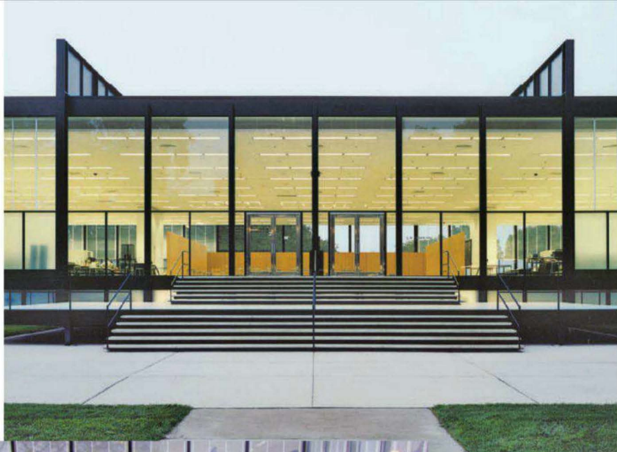
S.R. CROWN HALL, ILLINOIS INSTITUTE OF TECHNOLOGY, CHICAGO. MIES VAN DER ROHE, 1956. RENOVATED BY KRUECK+SEXTON ARCHITECTS, 2005.
