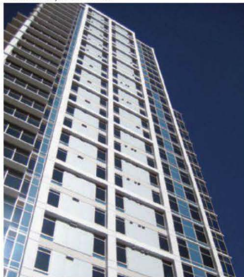
The Sapphire Towers in San Diego have glazed openings with a minimum 45-minute fire rating.
