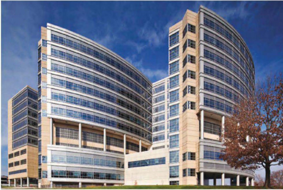
The University of Michigan C.S. Mott Children's Hospital and Von Voigtlander Women's Hospital was designed by the firm HKS to use low-E glazing with low reflectivity and a neutral appearance.
