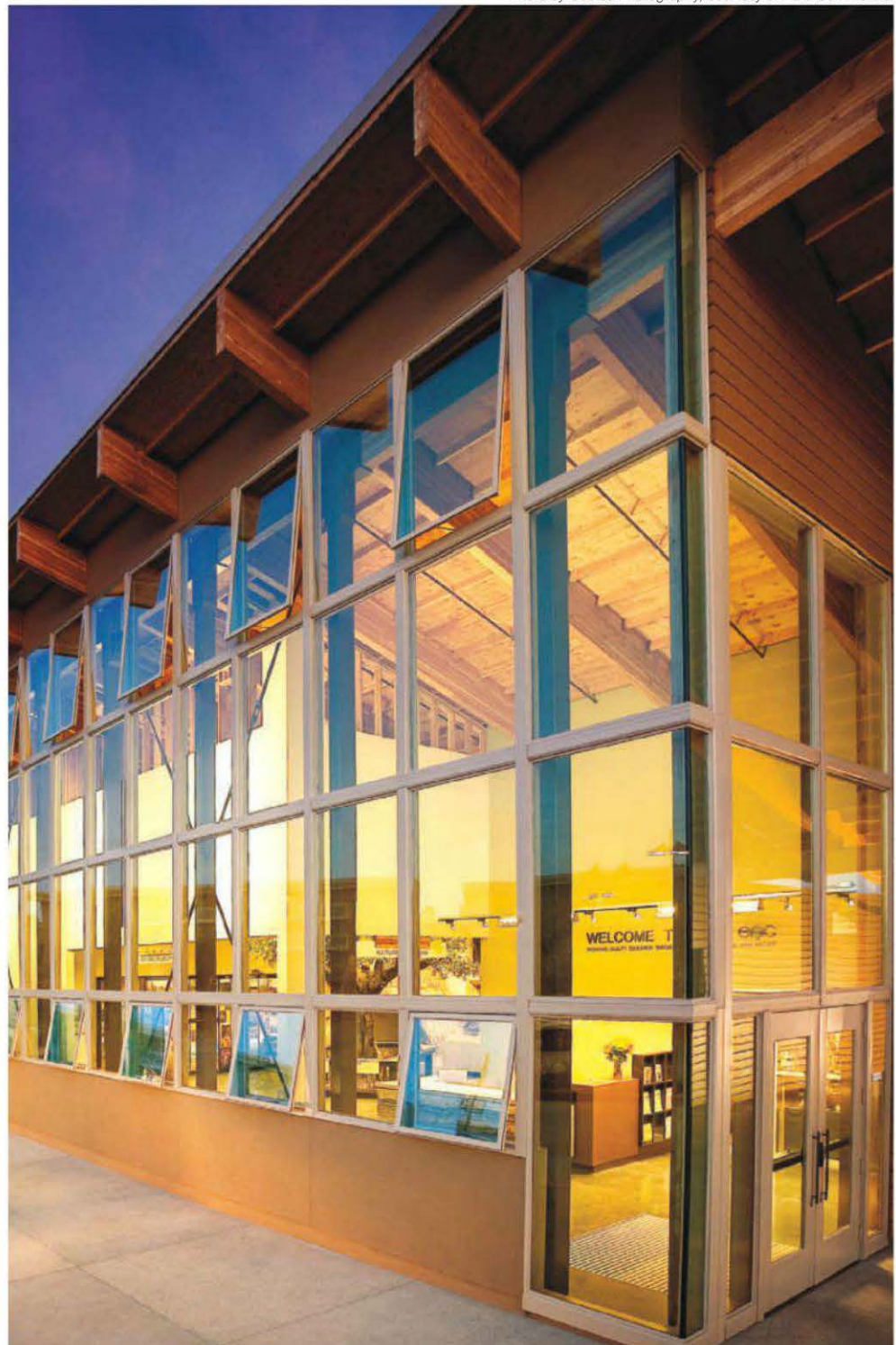
A high-performance aluminum-clad wood window wall at the Environmental Nature Center in Newport Beach, Calif., captures natural ventilation and daylight while limiting heat gain with advanced, low-E insulating glass.
