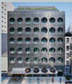
Handel Architects' Dream Downtown Hotel opened last year in New York City.
