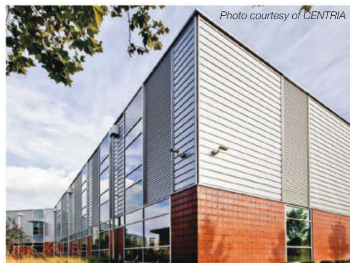
Designed by architect SRG Partnership, the Chemeketa Community College’s 74,000-square-foot project revamped the facilities that house space and equipment for nursing, dental hygiene and pharmacy technology students, with a durable metal-panel cladding system incorporating an insulated composite back-up panel.
