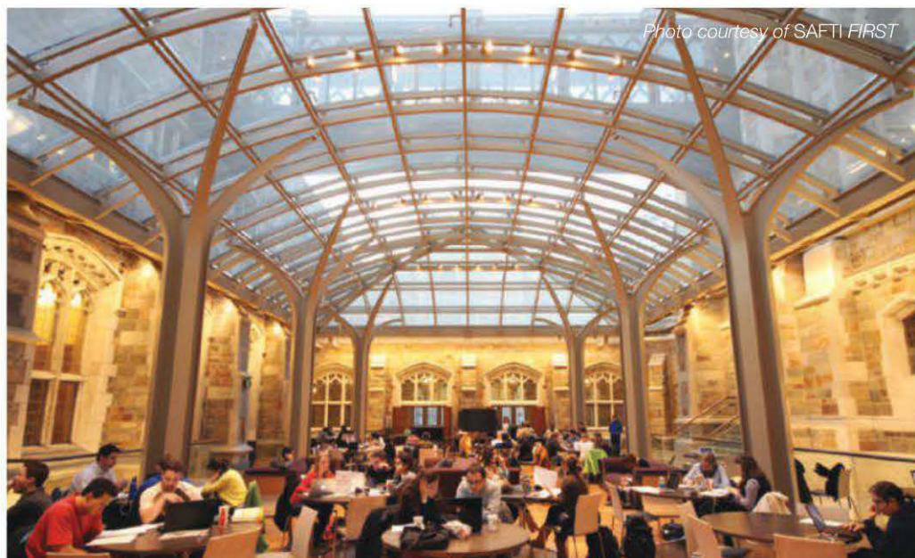
The University of Michigan Law School blended a historical restoration with a contemporary addition including a glazed space-frame canopy, designed by Huntman-Cox and Integrated Design Solutions. Stained glass windows in the 1933 limestone walls were mated with 2-hour rated fire-resistive glass panels to preserve the original look.
