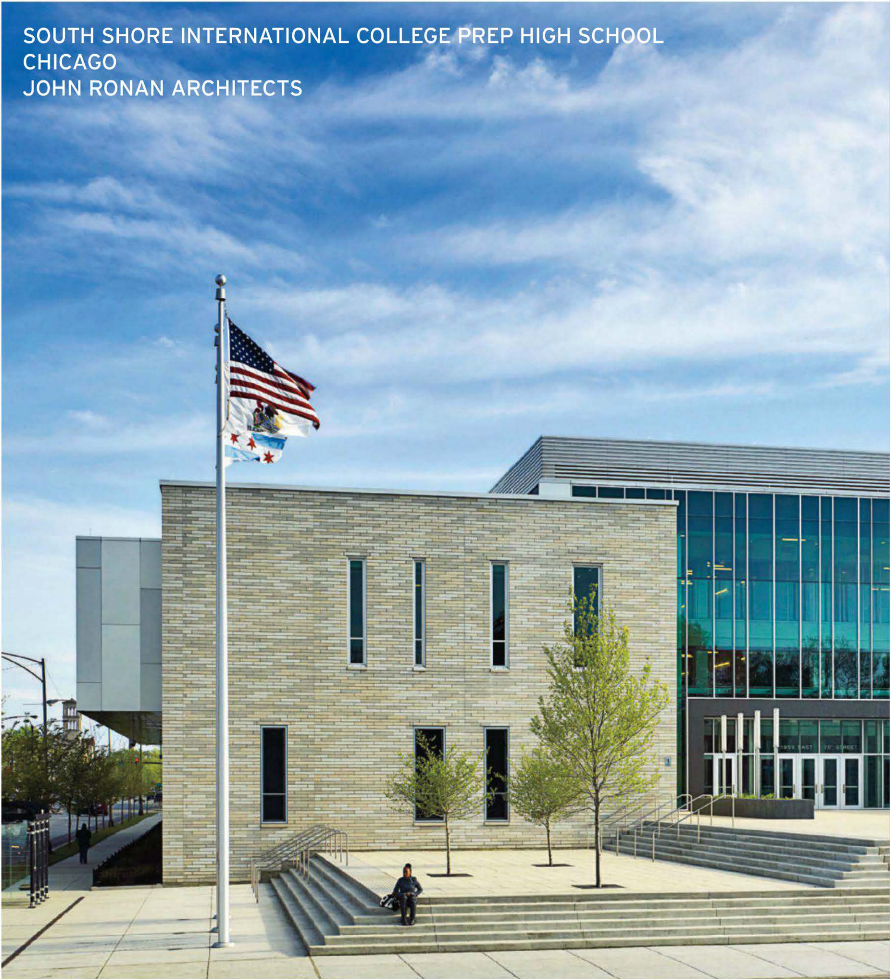
The high school's main entrance at the northeast corner is elevated on a plinth, which is intended to give the school a sense of importance as well as to provide sitting areas on the steps.
