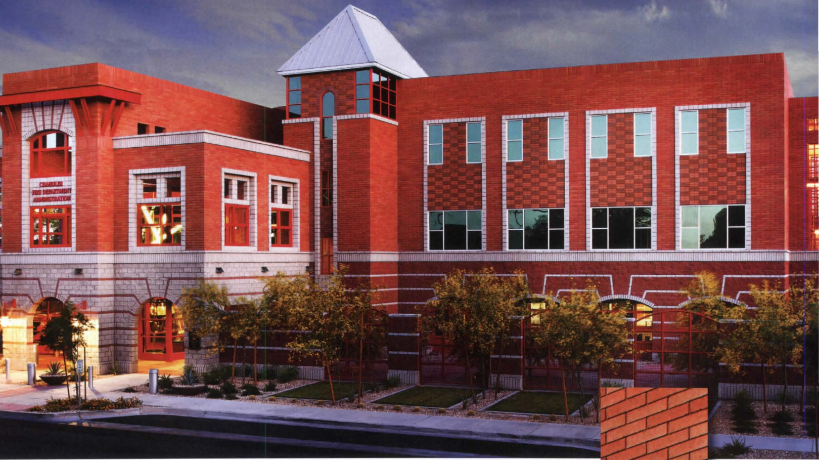
-Project: Chandler Fire Administration Building, Chandler, AZ.
