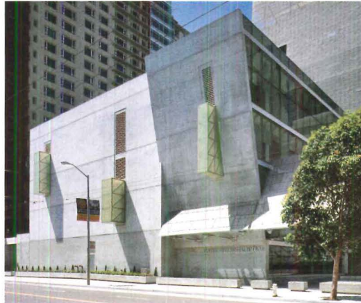
LEFT: The four-story barlike annex terminates with a sculptural end elevation on Mission Street.
