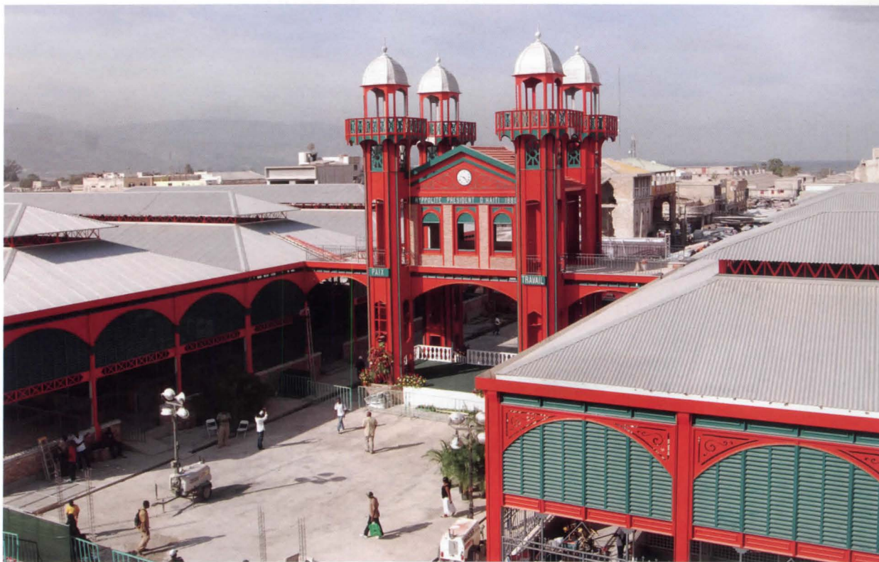
Architect John McAslan has revived the Iron Market (above), which suffered extensive damage during the 2010 earthquake (below).
