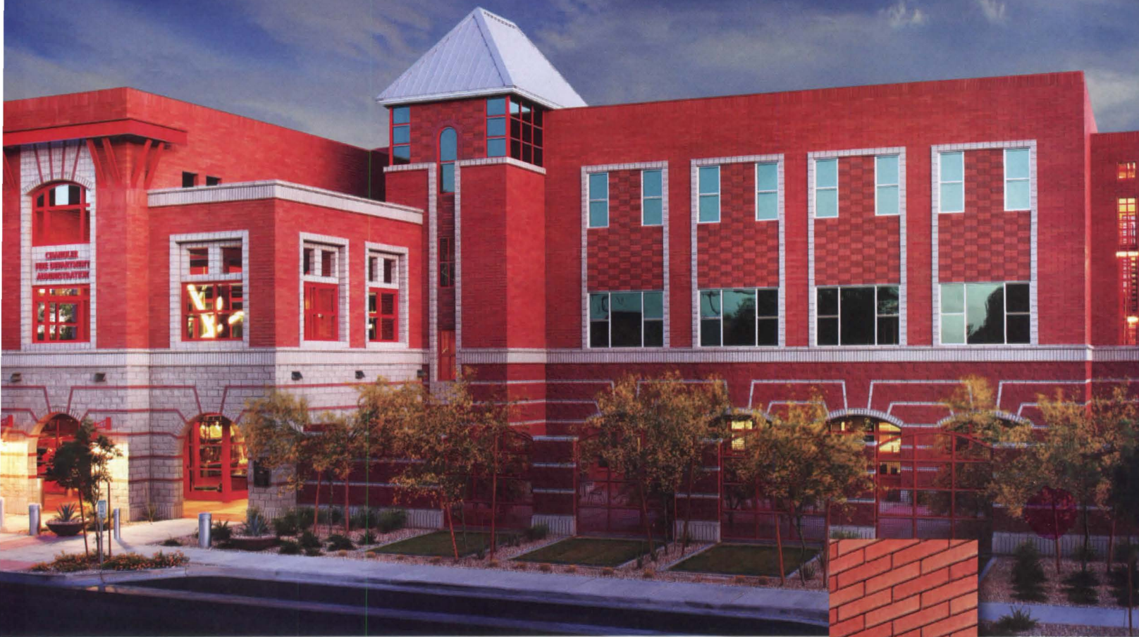
-Project: Chandler Fire Administration Building, Chandler, AZ.
