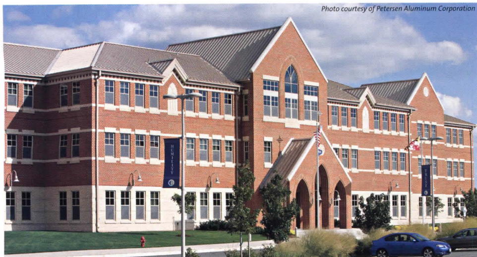
Standing seam metal roofs bring new aesthetics to school designs.
