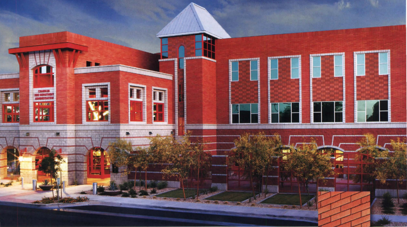
-Project: Chandler Fire Administration Building, Chandler, AZ.
