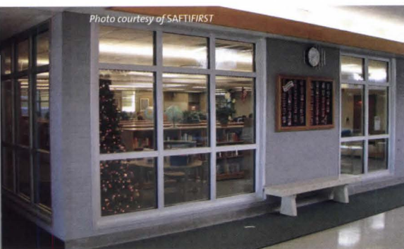
Stringent fire-safety criteria were met in the corridor designs at North Layton Junior High School.
