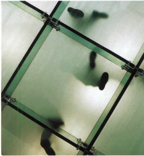
Without the use of highly transparent low-iron, or white, glass, the walkway has a greenish tint.
