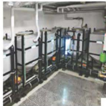
1. A rendering of the Pontos AquaCycle 2500, showing the unit's three 200-gallon tanks made of high-grade polyethylene. 2. The system comes in a range of model sizes that can be adapted to meet almost any demand, from 600 to 15,000 gallons per day.
